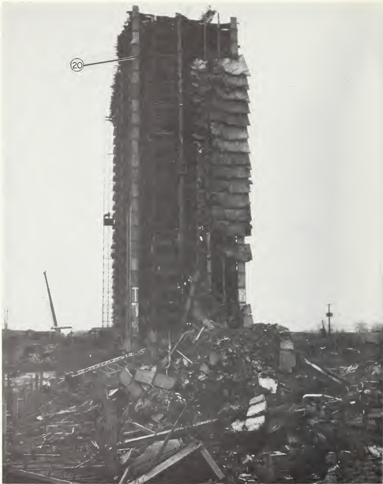
Figure 2.13 Appearance of A-4 after the removal of the east end of the building, viewed from the east.
