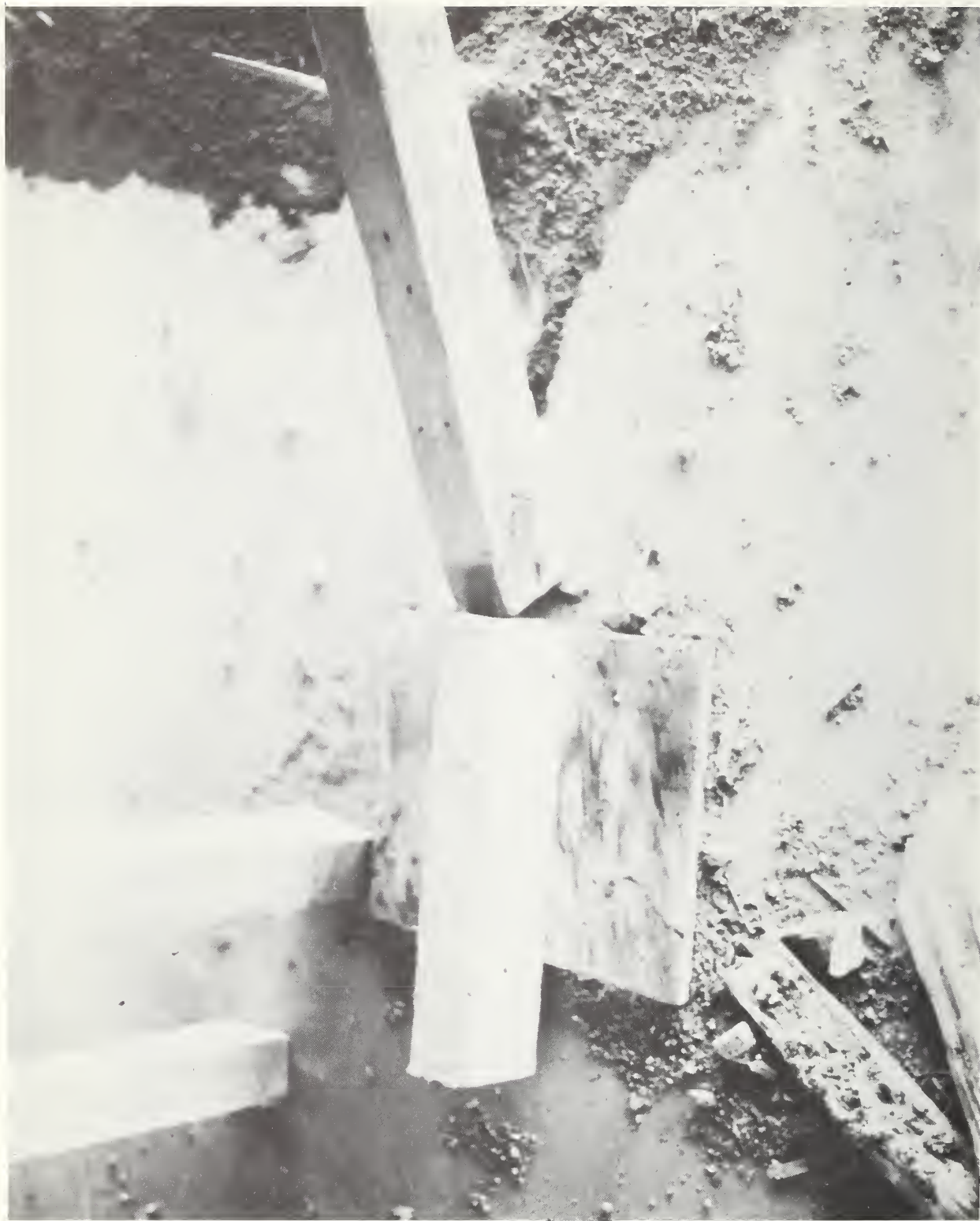
Figure 2.21 Detail at base of lateral bracing, 23rd floor.
