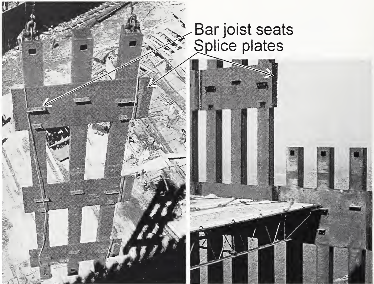
Figure 2–17. Perimeter column wall panel and steel truss floor modules.
