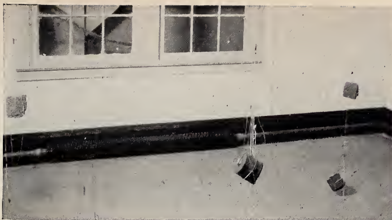
FIGURE 5. Baseboard convector without the sheet-metal enclosure showing the method of installing the connecting pipes.
