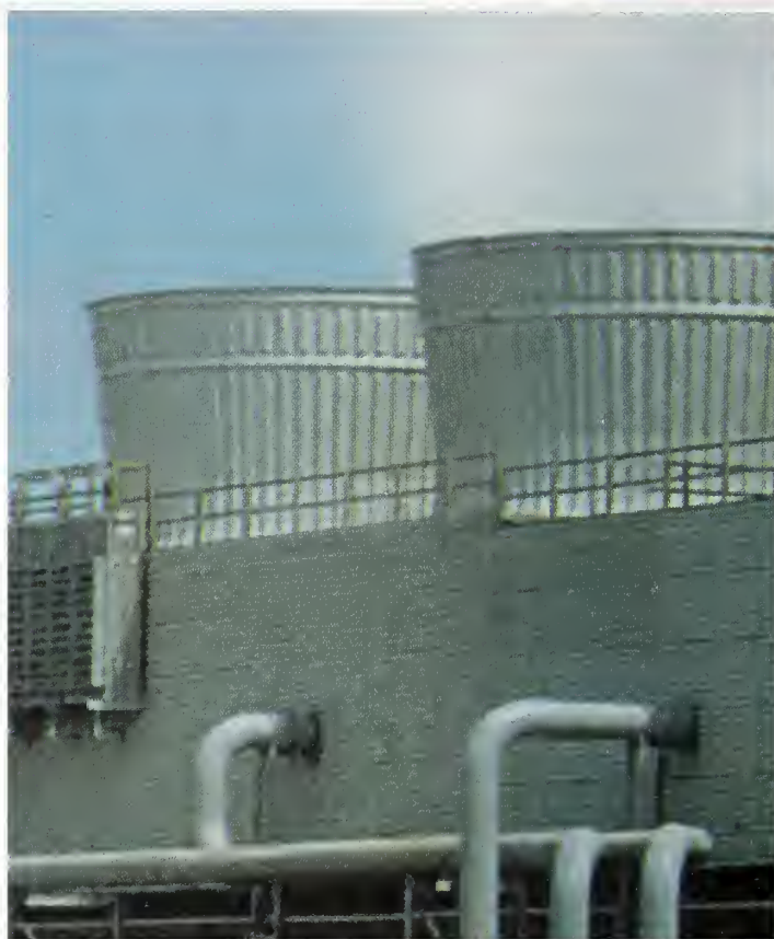
FIGURE 1. No discernible cloud is emitted by the plume-abated cooling tower shown on the left compared to the plumes emerging from the non-abated towers on the right.
