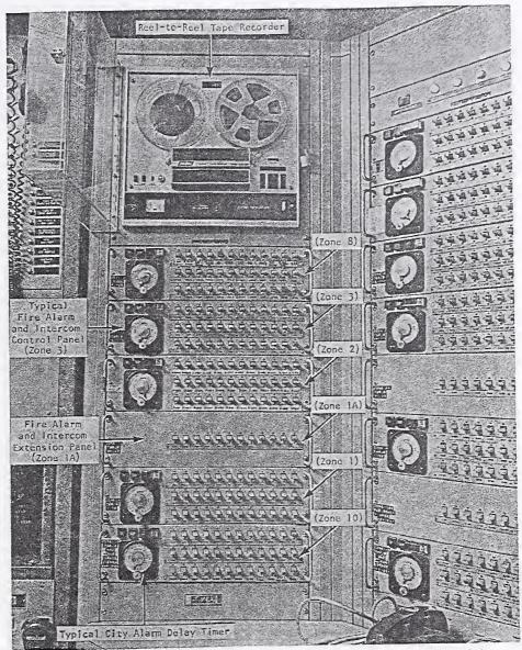
Figure 3-5. Fire alarm console (Zones 1, 2, 3, 8, 10).
