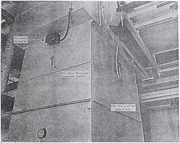
Figure 3-9. Typical return air duct and duct detector.
