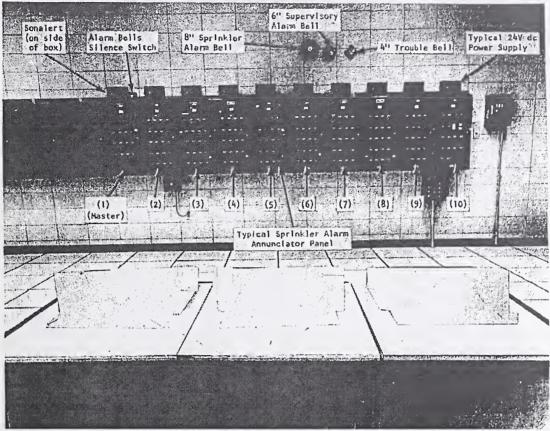
Figure 3–16. Sprinkler alarm annunciator in HVAC computer room.
