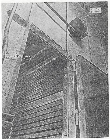
Figure 3-8. Typical supply air duct detector installation.
