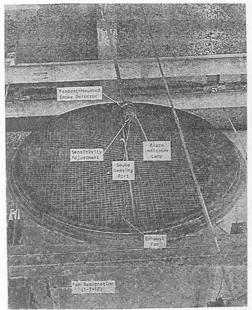
Figure 3-10. Typical pendant mounted smoke detector.
