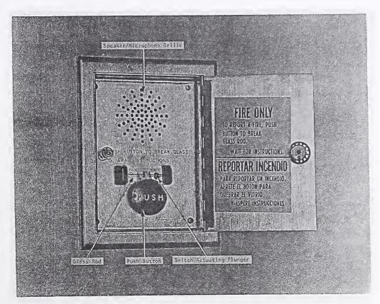
Figure 3–2. Interior of break-glass station.
