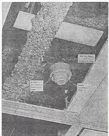
Figure 3–6. Typical interior return air smoke detector (ceiling tile removed).
