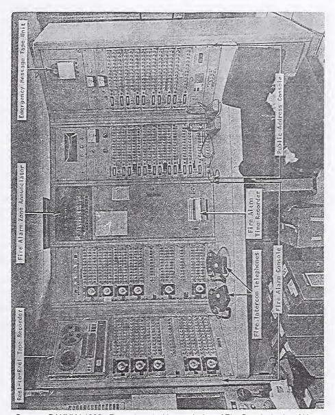
Figure 3-4. Fire alarm console.
