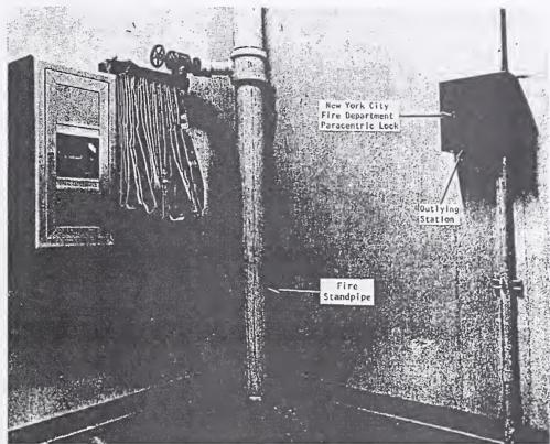
Figure 3-18. Outlying station of Standpipe Fireline Communication System.
