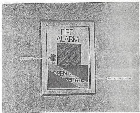
Figure 3-1. Typical break-glass station.
