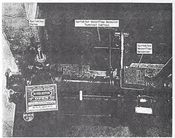
Figure 3–15. Sprinkler waterflow detector installation.
