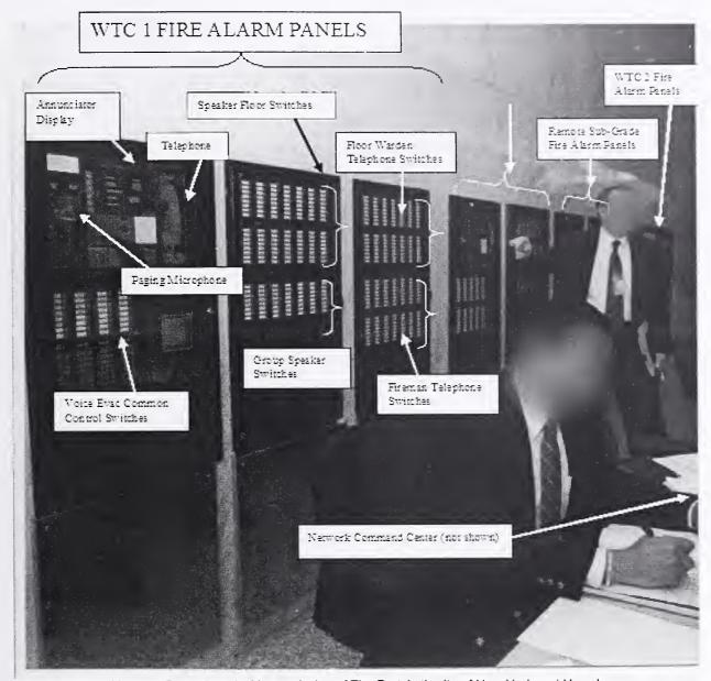
Figure 5–16. WTC 1 fire command station.
