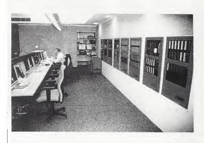
Figure 5–25. Operation Control Center located on the B1 Level below WTC 2 with redundant fire alarm system controls.
