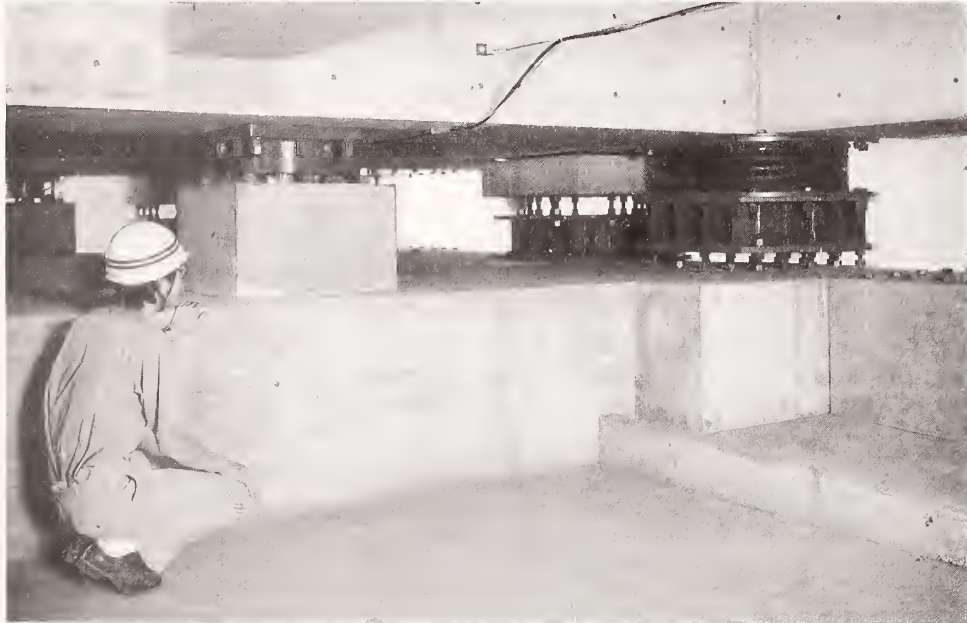
Various devices fitted at the foundation.
