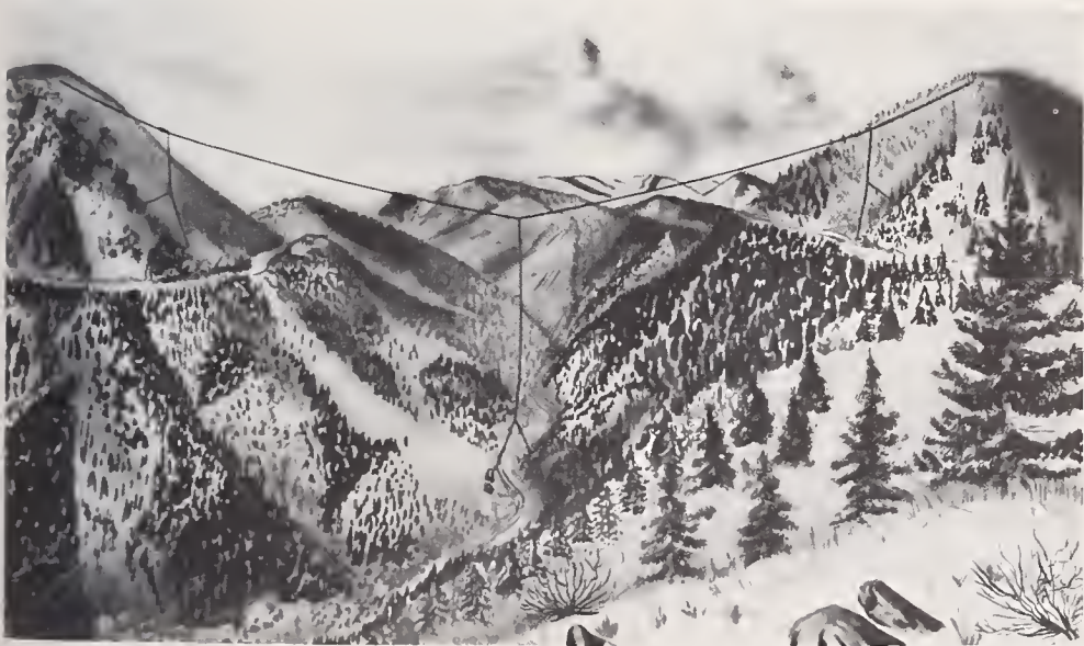
A new 20 kc/s standard frequency station was put into operation this year near Boulder, Colo. The antenna, a copper coated steel cable, weighs more than a ton, stretches 3,400 ft from anchor to anchor, and is 900 ft above the canyon floor (page 39).
