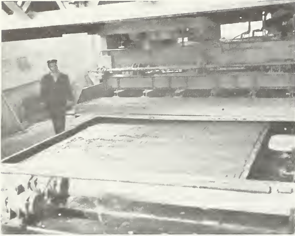
Moscow Conveyor, End Station: Form Stripping and Removal
