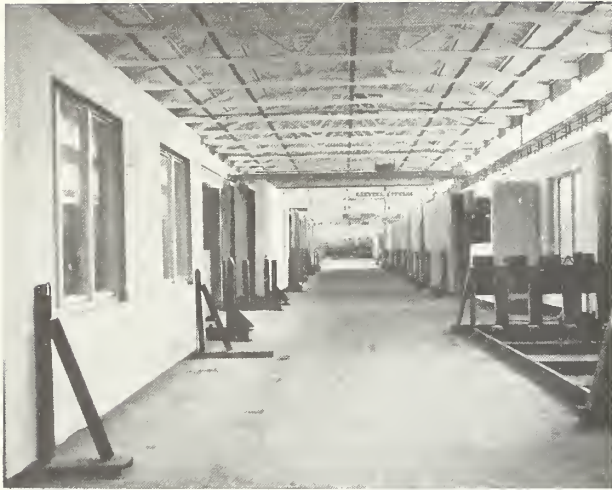
Leningrad: Finished Exterior Panels Await Transport
