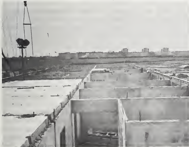
A Leningrad Project: Note Interior Panel Construction
