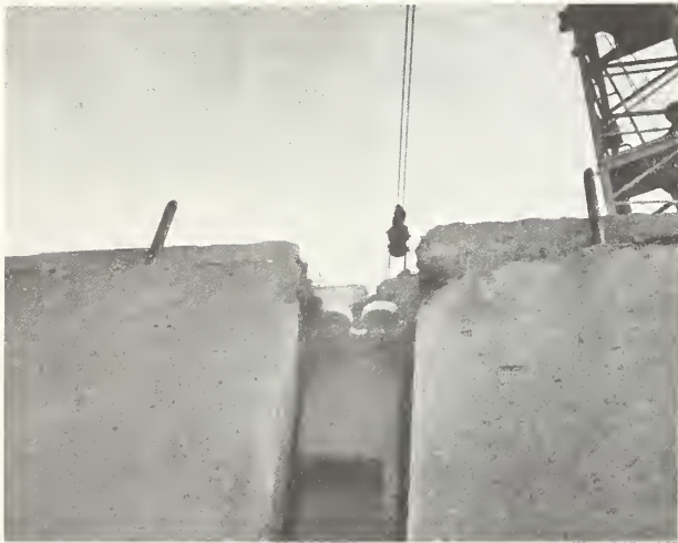
Pin and Socket Detail: Leningrad
