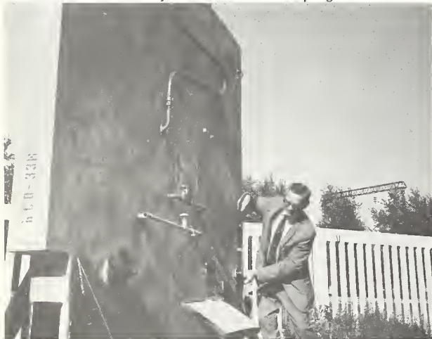
Moscow Exhibit: Utility Wall Panel with Piping Cast-in
