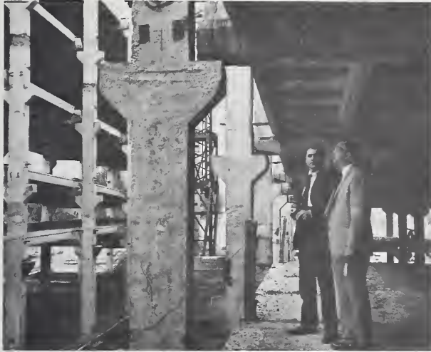
Kiev Taxi Garage: Girder Beam Connection
