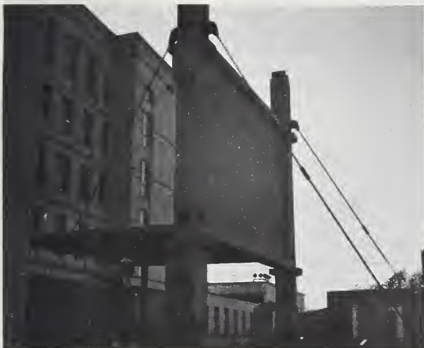
Moscow Exhibit: Precast Column, Deck, and Wall Assembly
