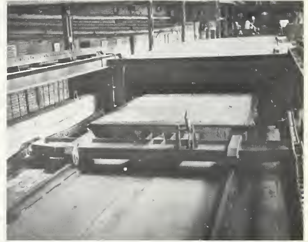
Moscow: Concrete Emerging from Curing Oven
