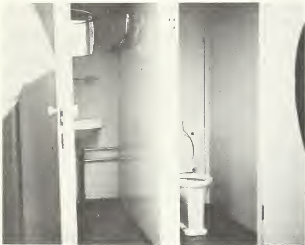
Kiev Bathroom Box: Hot Water Pipe Doubles as Towel Rack
