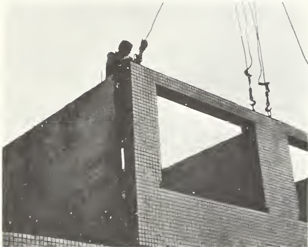
Leningrad: Exterior Wall Panel Erection
