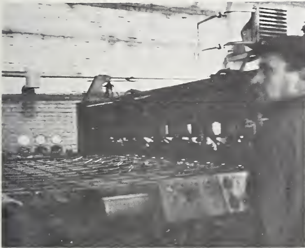
Kiev: Automatic Welder for Reinforcing Mesh
