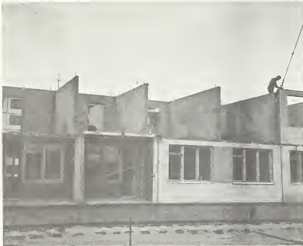
Leningrad: Placing Tiled Exterior Walls
