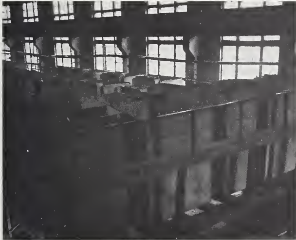
Bathroom Boxes Await Finishing: Leningrad
