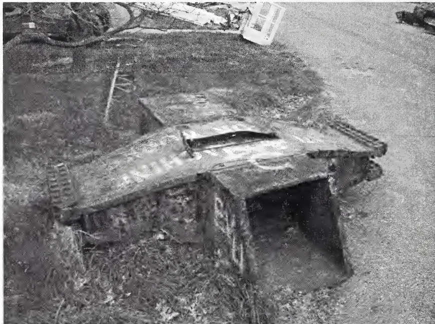
B-5004 portion cut and moved to NIST campus
