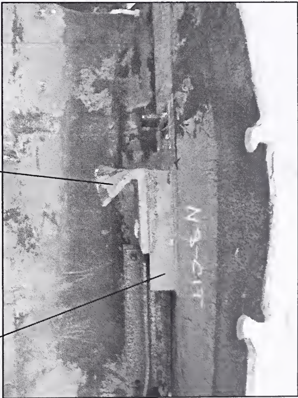
Figure A-2. Floor truss seats shown from sample N-8.
