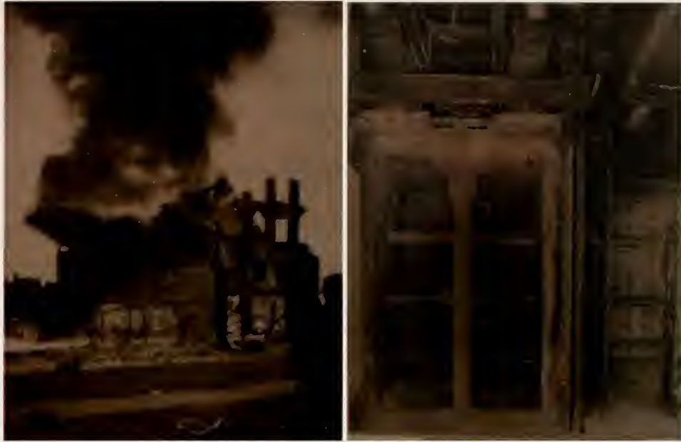
Figure 2 NBS Federal Triangle fire test (left) & NBS column furnace (right), 1920s.
