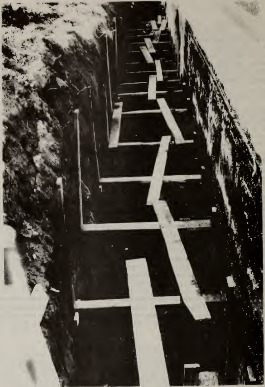
FACING PAGE: Spot bracing in dense clayey silt
