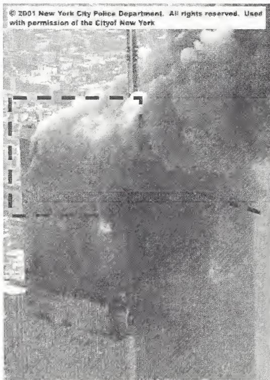
Figure 7–3. Impact damage to north and west faces of WTC 1.
