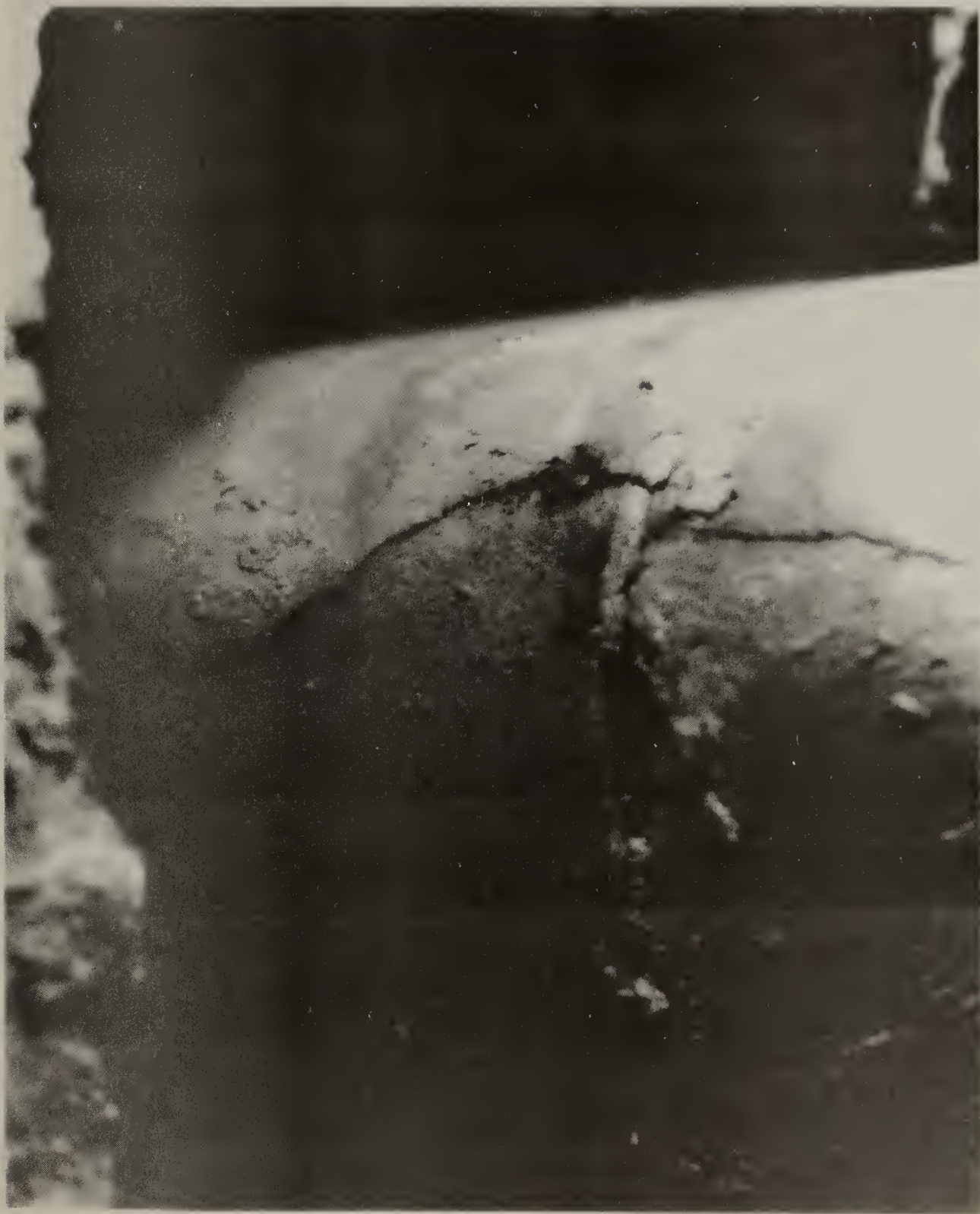
Figure 60. Damage to Masonry Chimney 3 After Chimney Fire.
