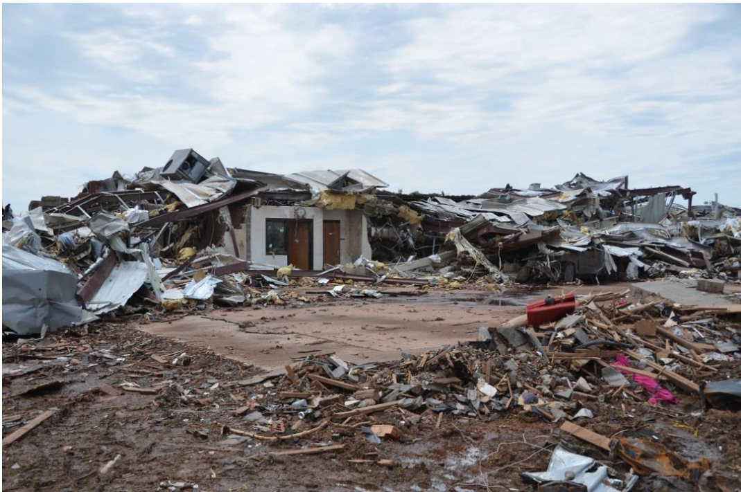
Figure 4-9. Collapsed Gymnasium building (Note the interior Gymnasium Office surrounded by a reinforced CMU wall remained standing).
