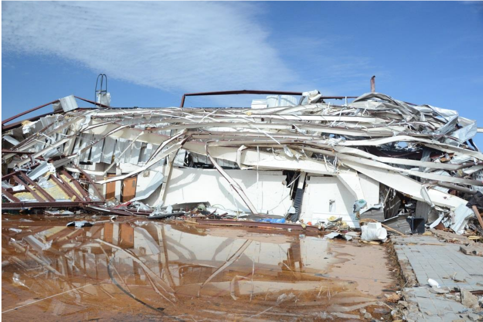
Figure 4-14. Collapsed Multipurpose Building of Briarwood Elementary School.
