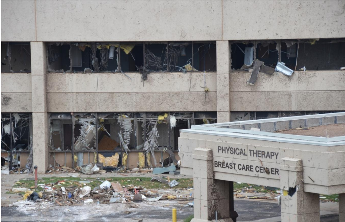
Figure 4-26. Damage to the envelope of Moore Medical Center (glazing).
