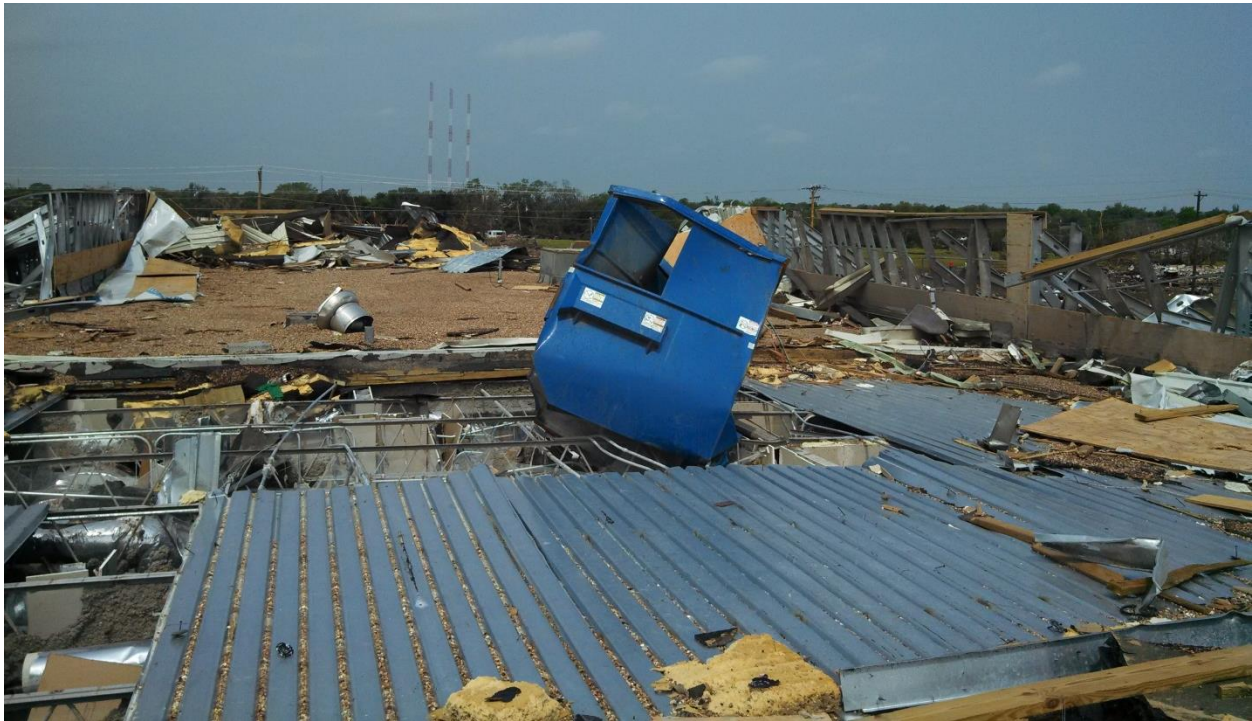
Figure 4-28. Impact damage to hospital roof bar joists from steel trash dumpster, and loss of steel roof decking.
