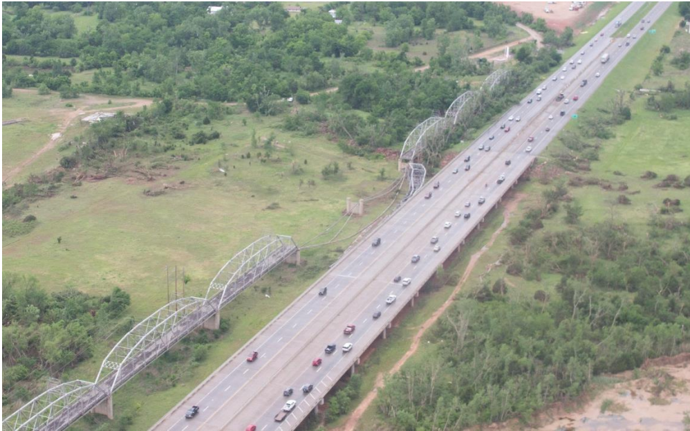
Figure 2-5. Two spans of the historic trestle bridge on US 62 running parallel to I-44 were destroyed. The bridge had been closed to traffic since 1963 but carried water pipes across the Canadian River.
