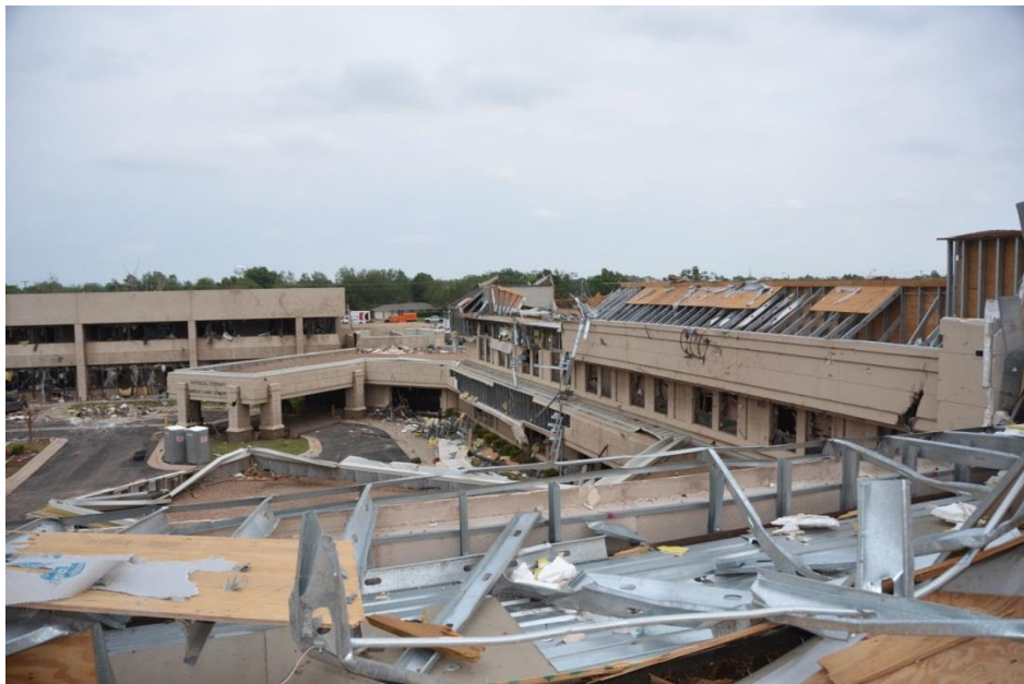
Figure 4-25. Damage to the building envelope and rooftop architectural elements of Moore Medical Center.
