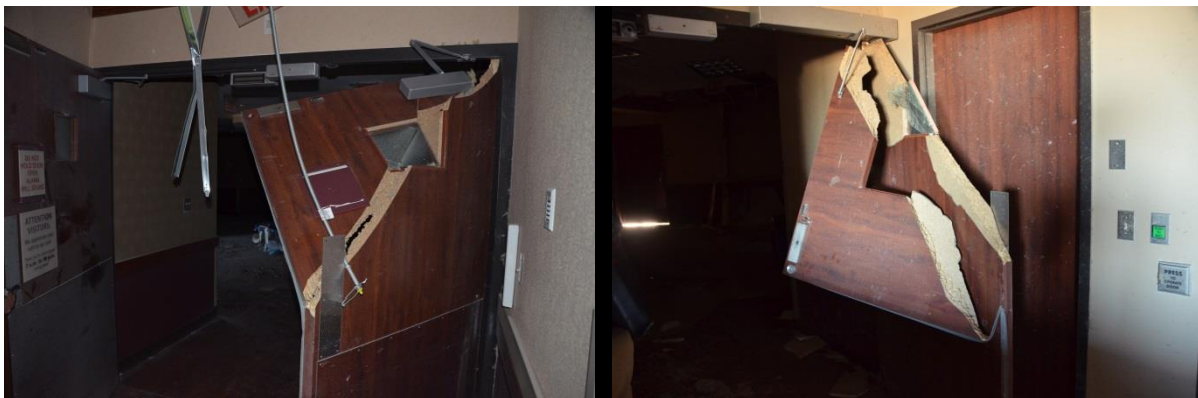
Figure 4-29. Examples of broken interior doors at the Moore Medical Center.
