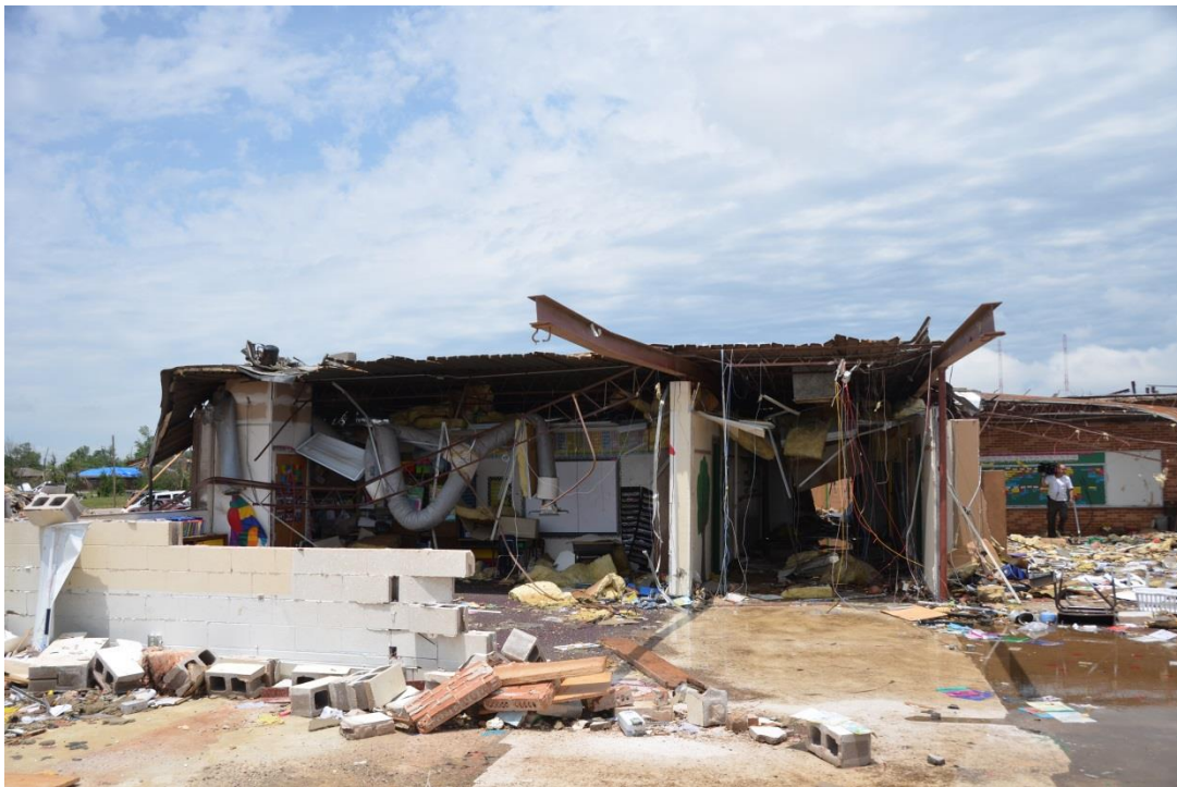
Figure 4-7. Collapsed southwest wing of original main classroom building.
