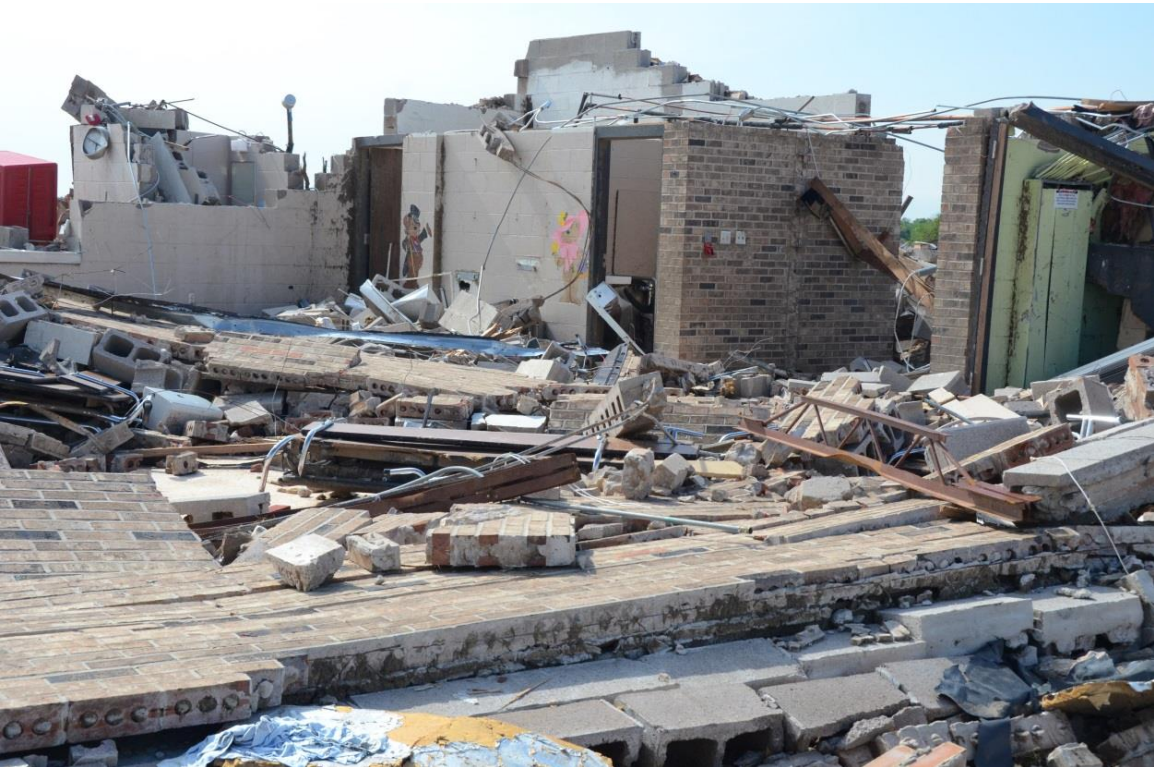
Figure 4-17. Cafeteria. Complete structural failure with only the interior bathroom remaining standing.
