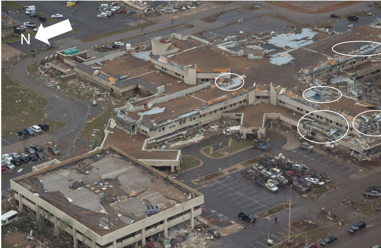
Figure 4-24. Aerial view of the heavily damaged Moore Medical Center (looking south-east). Circled locations indicate areas of roof deck damage.
