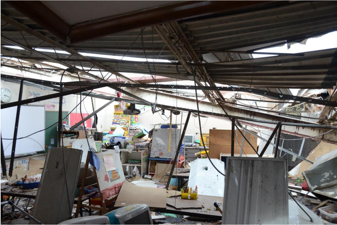
Figure 4-18. An interior view of a classroom in the 400 Building where portion of the building's metal roof system was lost.
