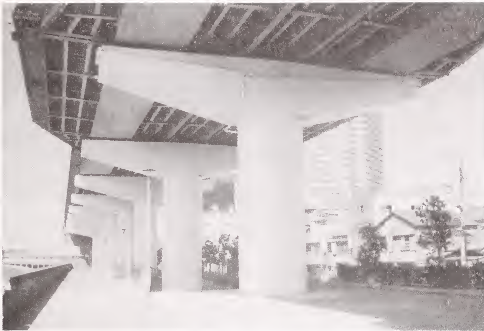
Photo 6 Seismic Strengthening of RC Piers on Metropolitan Expressway by Steel Jackets
