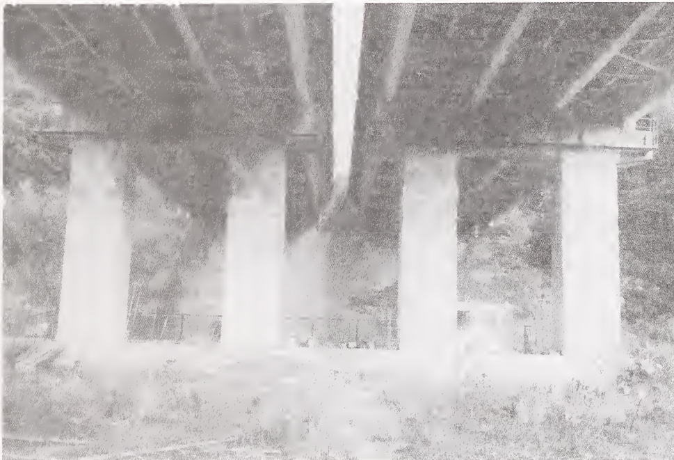
Photo 1 Seismic Strengthening of RC Frame by Placing New Reinforced Concrete
