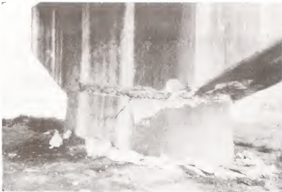
Photo 3 Damage of Sendai Bridge during Miyagi-ken-oki Earthquake in 1978
