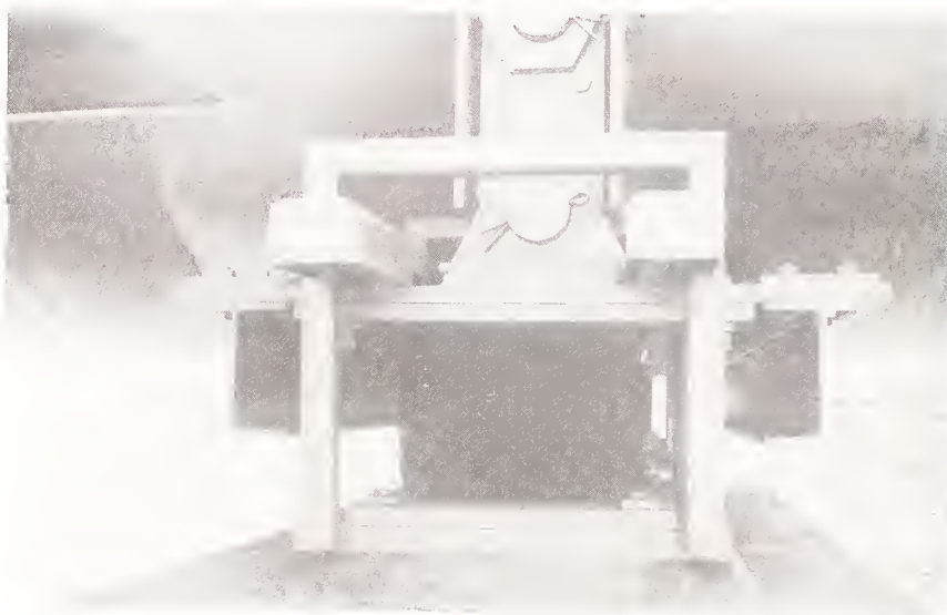
PIPE SUPPORT BEARING AND BEARING STOP - FIGURE 8
