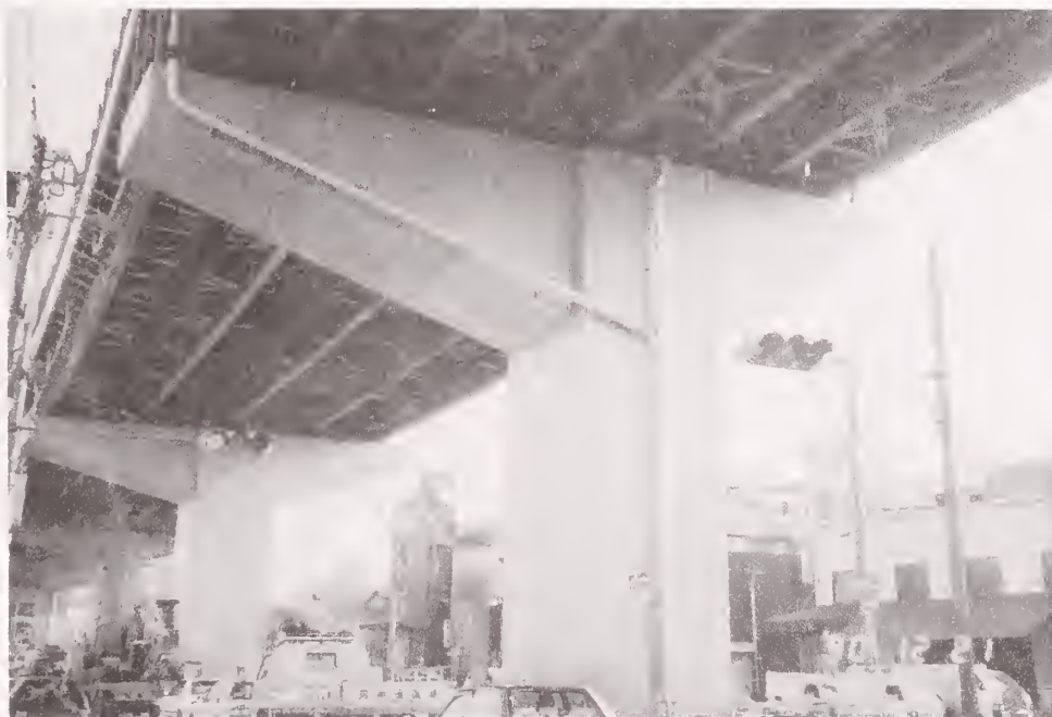
Photo 7 Seismic Strengthening of RC Piers on Hanshin Expressway by Steel Jackets
