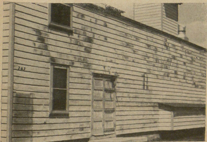
FIGURE 10.— Typical discoloration of paint due to mildew. Before repainting, surface should be scrubbed with water containing some alkaline cleaner, for example, trisodium phosphate.
