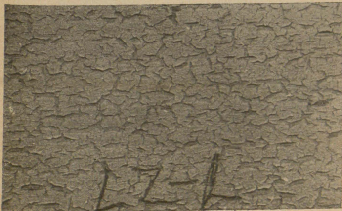
FIGURE 30.— Alligatoring of paint on fence.
