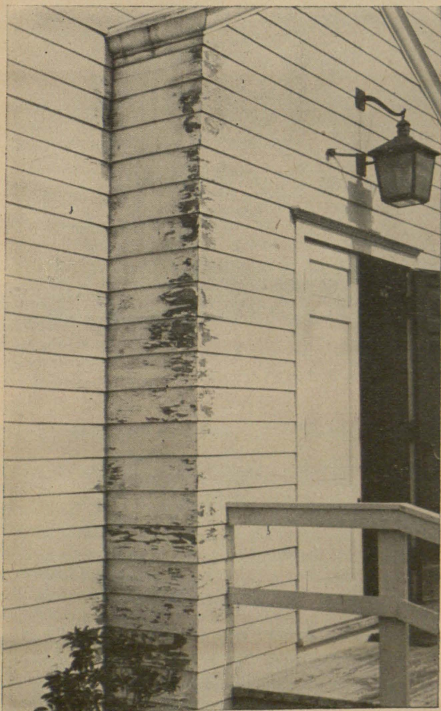
FIGURE 18.— Serious peeling of paint.
