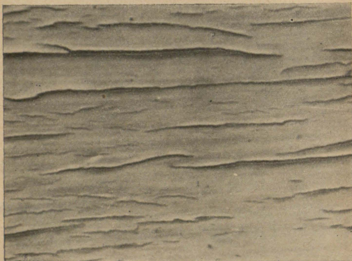
FIGURE 19.— Details of paint cracking on exterior of wood building.
