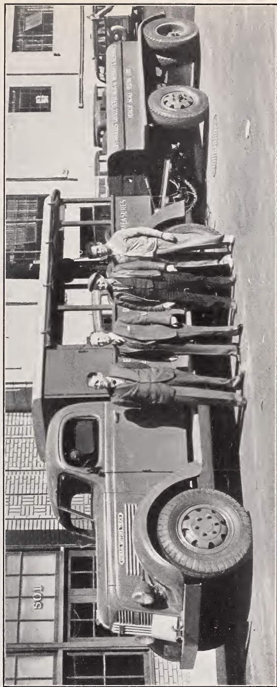
FIGURE 11.—General view of large-capacity scale-testing equipment of Los Angeles County, California, showing steel trailer standardized at 20,000 pounds.
