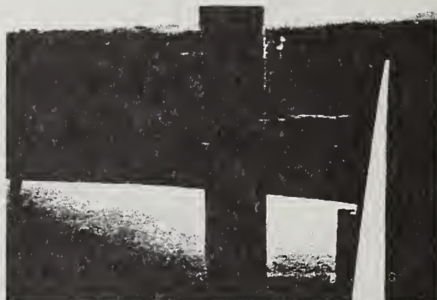
Photo 4 Depressed levee at the right bank downstream of the Yokotone Gate
