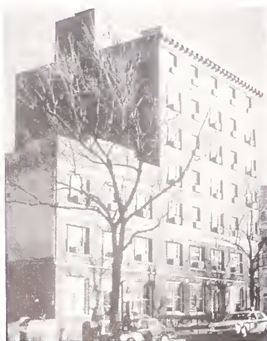
Figure 13. Plaza Hotel in Washington, DC, unoccupied at the time, in which fire experiments were conducted.
