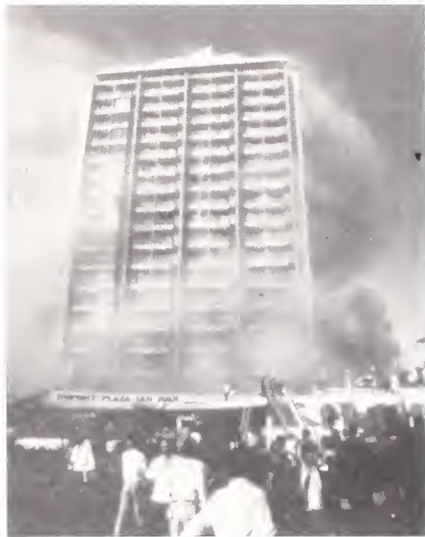
Figure 3. Dupont Plaza Hotel fire, San Juan, Puerto Rico. Reprinted with permission from NFPA [4].
