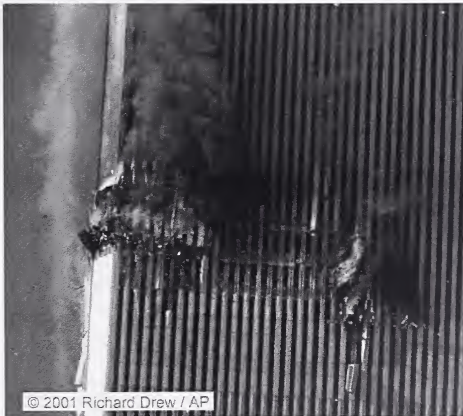
Figure 9-126. Impact Damage to the Northeast Corner of the Exterior Wall of WTC 2.
