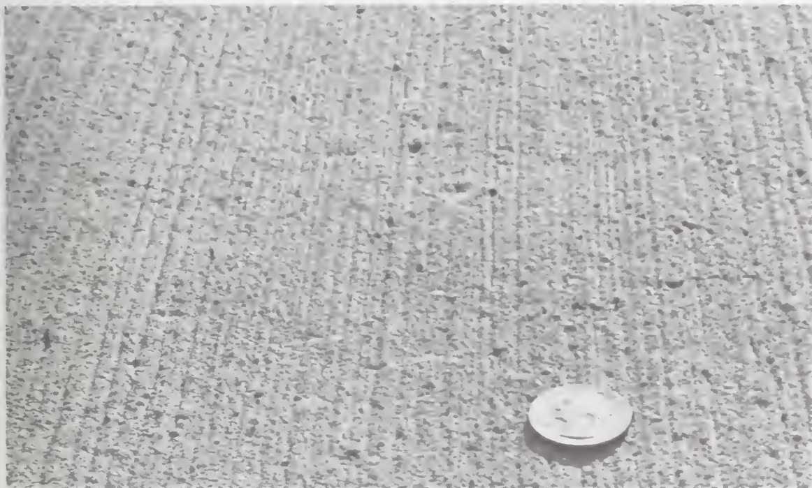
Figure 8. Continuous poured reinforced concrete surface on Interstate-81 near Carlisle, Pennsylvania. Traffic flow would be from left to right.
