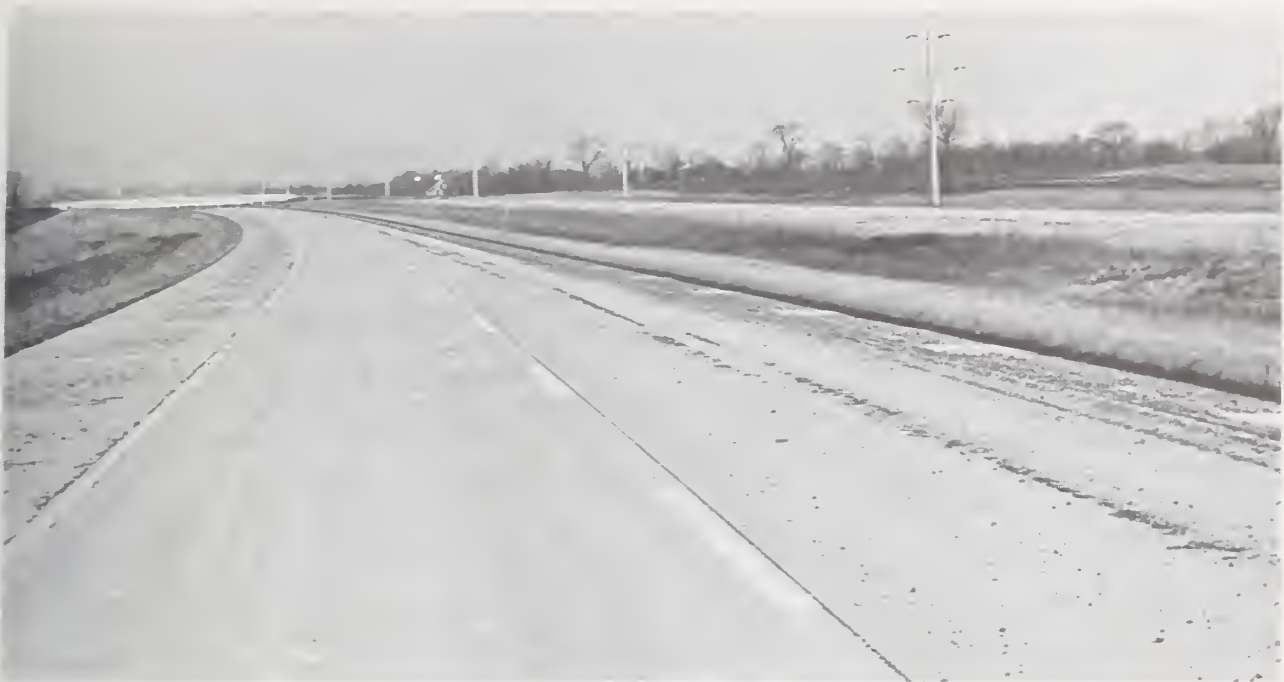
Figure 7. View of continuous poured reinforced concrete test section looking northeast.
