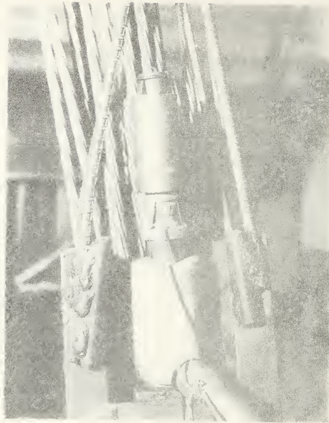
Figure 2.25 Pre-tensioning loading tendon strands
