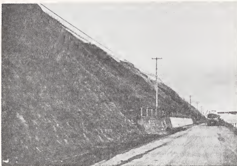
Photo. 3 Light Damage to Slope along National Highway Route 235, at Irifune Area, Shizunai Town. Retaining Walls Protected from a Large Failure.
