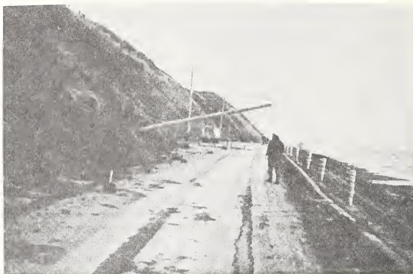
Photo. 1 Damage to Slope along National Highway Route 235, at Irifune Area, Shizunai Town. An electric post was overturned.
