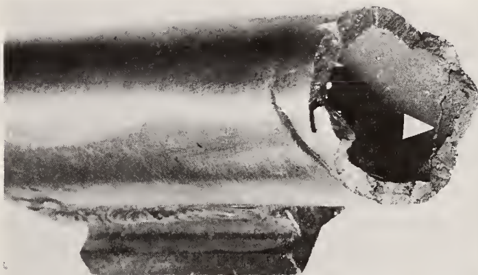
FIGURE 3. SCC in 1 in diameter superheater tube made of AISI type 347 stainless steel. The corrodent may have been chloride in "carry-over", concentrated by evaporation. The stress responsible for cracking is presumably due to a bending moment generated by thermal stresses and the support shoe (bottom) frozen in place by fly ash. Eighteen out of forty-five such superheater tubes failed thus in ninety steaming hours. Careful attention to boiler water chemistry to diminish carry-over solved the problem.
