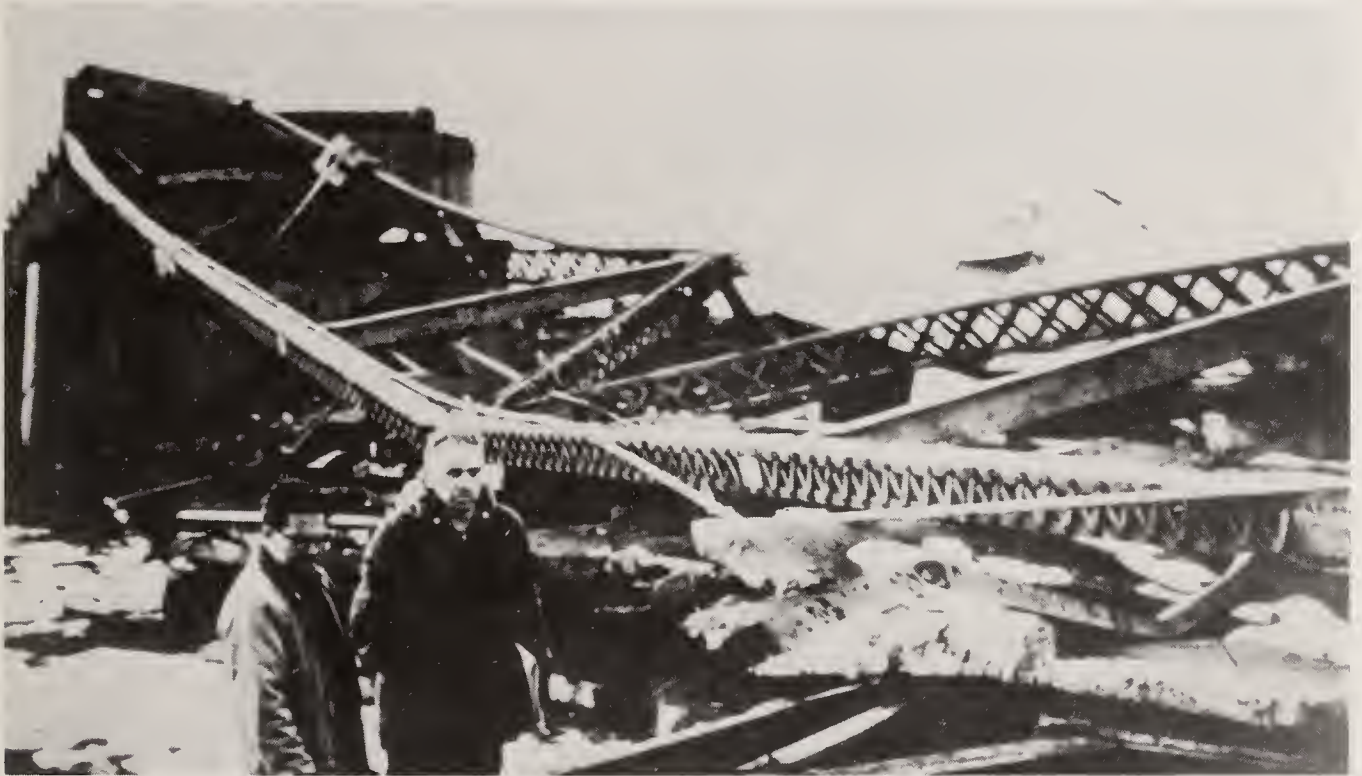
Consequence of stress corrosion cracking in a nonredundant load path structure: collapse of the "Silver Bridge" over the Ohio River, which occurred on December 15, 1967, carrying 46 persons to their death. Photo courtesy of Mr. H. C. Burnett, National Bureau of Standards.
