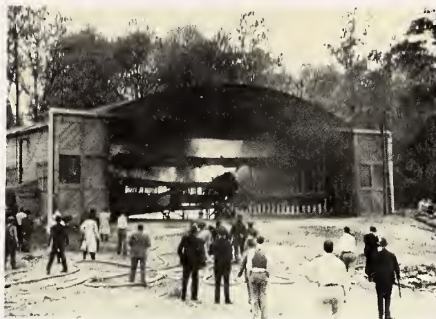
The Bureau became involved in fire-resistance testing early in its history. Shown above is testing performed on automatic sprinkler systems for airplane hangers in the 1930's. At the left, Randall Lawson demonstrates the test used today to evaluate the ease with which materials will ignite.
