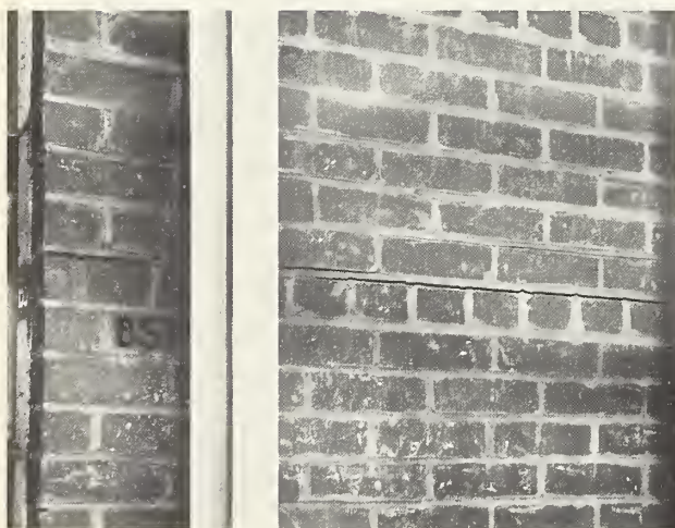
FIGURE 24. Flexural bond failure above header course in brick facing of composite wall.
