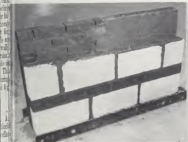
FIGURE 2. Composite wall under construction.
