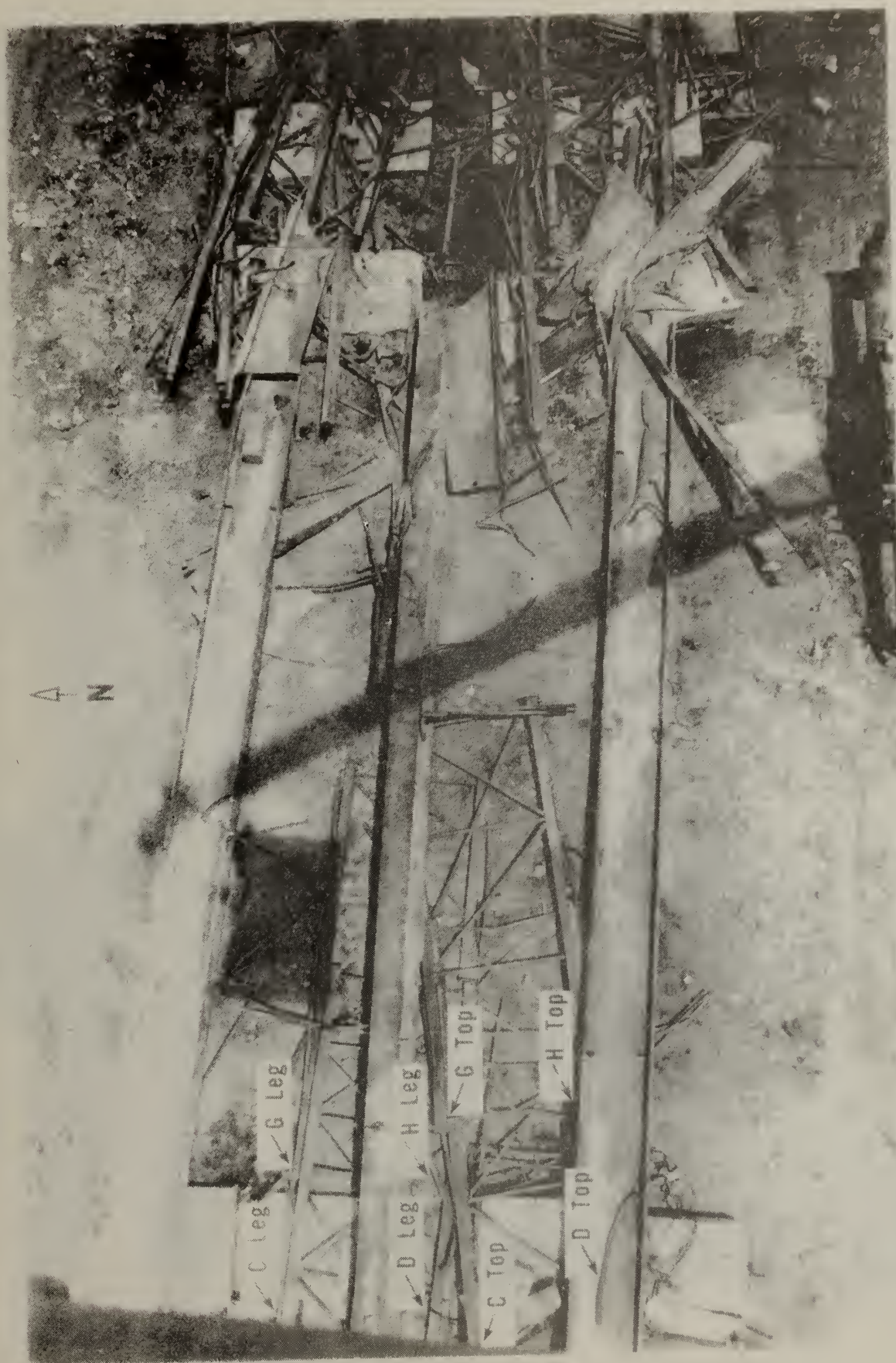
Figure 3.20 Location of parts of the south tower at 407.1
