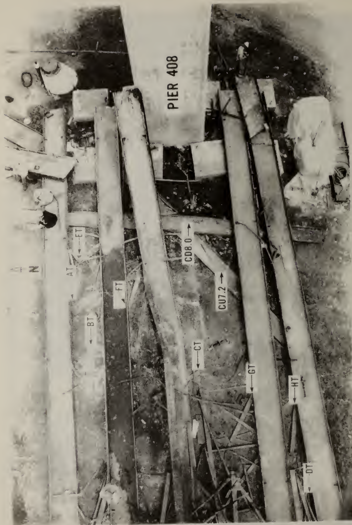
Figure 3.19 Location of the top sections of the shoring towers at 407.2
