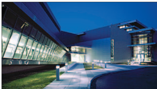
Figure 1. The CNST is located in the NIST Advanced Measurement Laboratory Complex, including the NanoFab cleanroom seen on the left. (Photo courtesy HDR Architecture, Inc./Steve Hall © Hedrich Blessing.)
