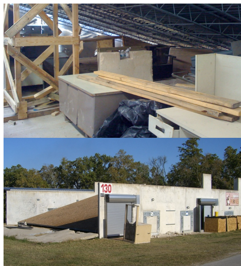
Figure 5: House of pancakes training scenario simulating a partially collapsed concrete building. The top picture shows the main area inside with the collapsed sloped roof and the bottom picture shows the building from the outside.
