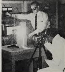
The demand for improved high-temperature materials has put special emphasis on the study of the properties of materials at high temperatures. Typical NBS studies include the melting behavior of ceramics (right), and the effects of high temperatures and high pressures on crystallization (left).
