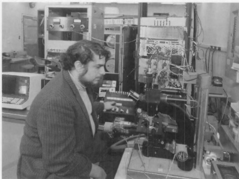
Phillip Stein of the NBS Center for Computer Science and Technology viewed a slide through a computer-controlled microscope that he developed in collaboration with the National Institutes of Health in 1969.
