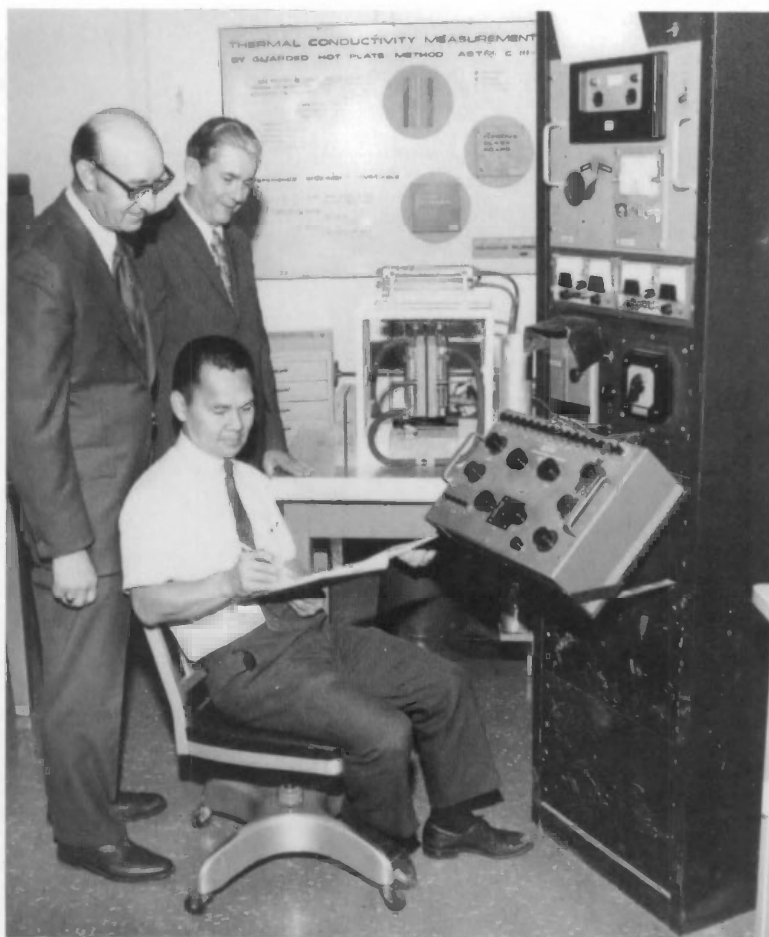
Frank J. Powell (standing on the left), Chief of the NBS Thermal Engineering Systems Section, and section colleague Thomas W. Watson watched as the Bureau's Chock I. Siu operated a guarded hot-plate apparatus (on table) to determine the thermal conductivity of insulation.
