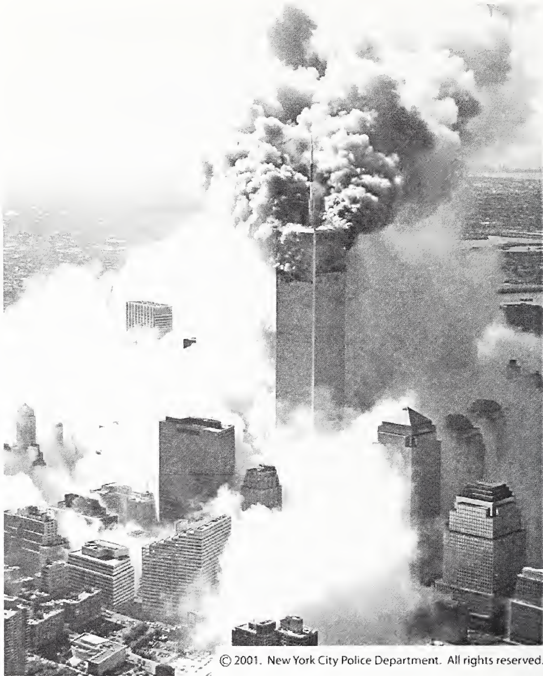
Figure 9–1. Collapse of WTC 2, viewed from north.
