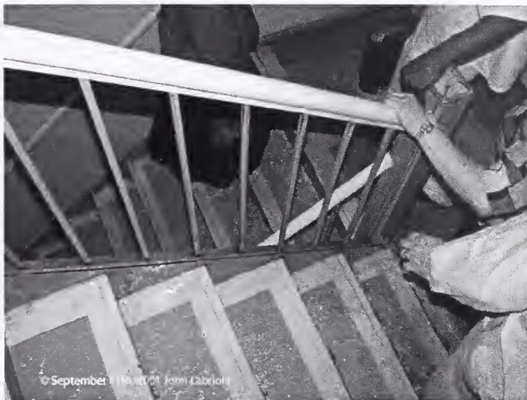
Figure 2–10. 44 in. stairwell in WTC 1 taken on September 11, 2001.
