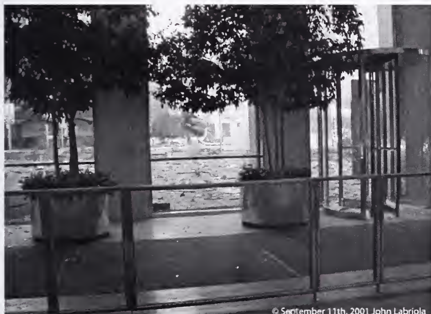
Figure 8–1. View from mezzanine level in WTC 1 looking east across WTC plaza, covered with debris. ‘Sphere,’ artwork by Fritz Koenig, can be seen on the plaza.
