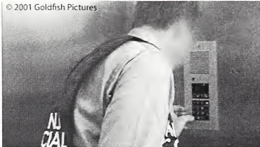
Figure 2–16. Elevator communication panel in the fire command station of WTC 1, as operated on September 11, 2001.
