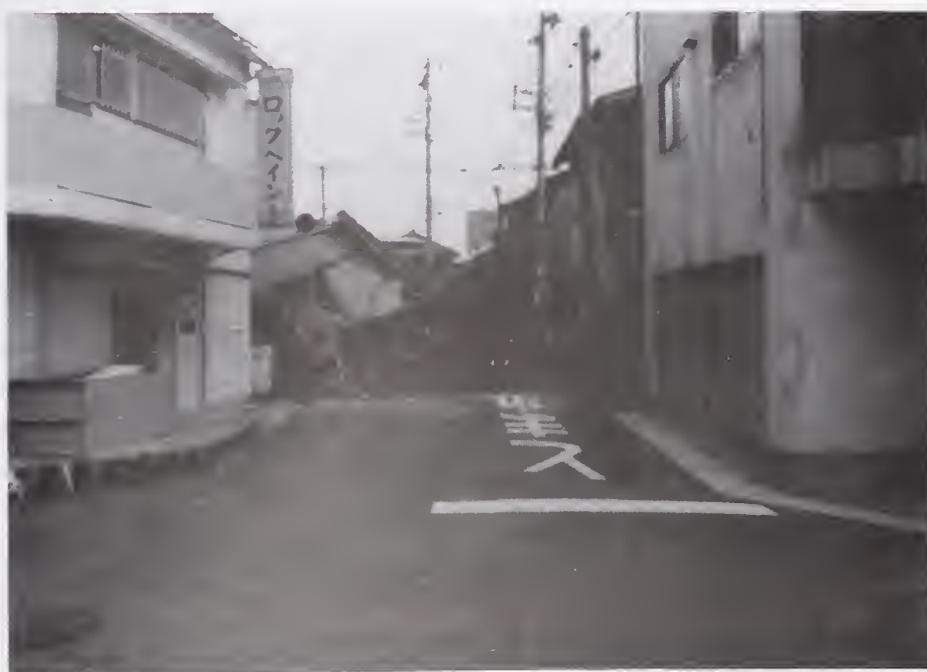
Figure 6.2.10 Collapsed structure across street.
