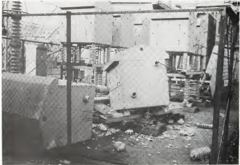
Figure 5.4.58 Neutral resistors failed, a device not used in this configuration in the U.S.
