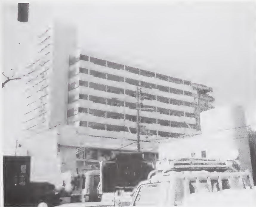
Figure 3.4.18 Fourth story collapse in apartment building.
