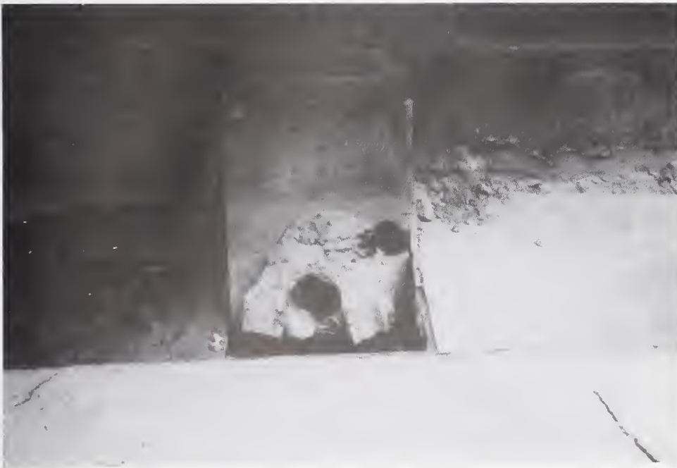
Figure 5.5.11 Settlement of a walkway adjacent to a building shears conduit and cables.
