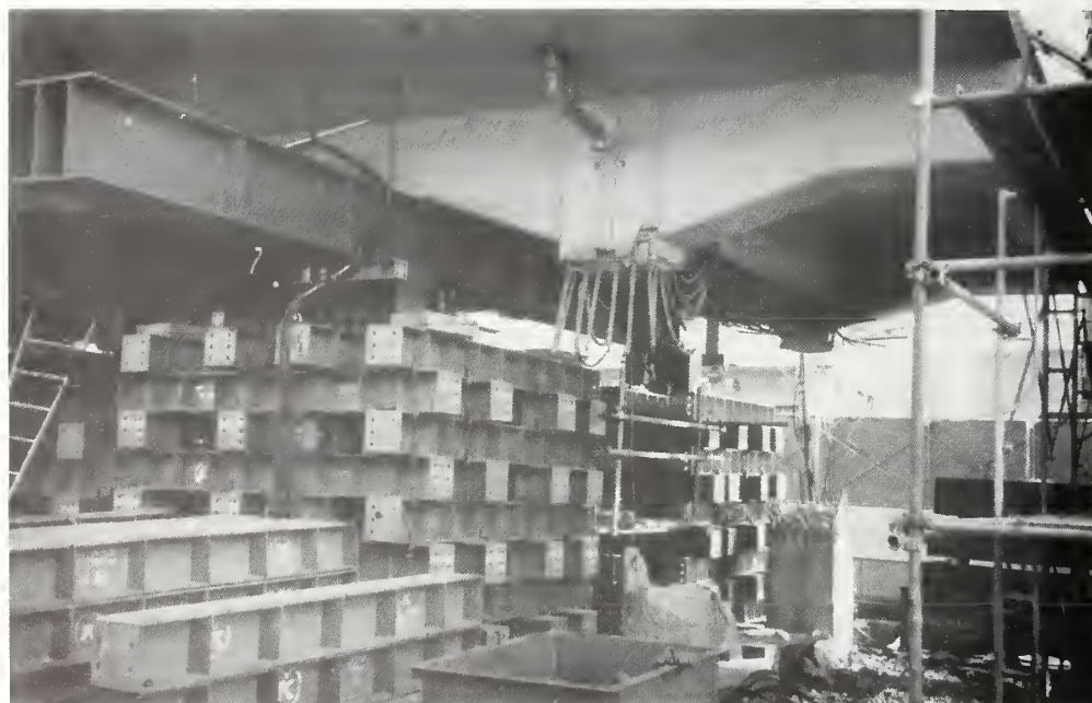
Figure 4.3.6 Column repair - Shinkansen.
