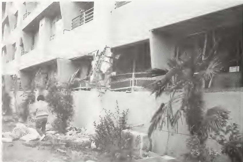
Figure 3.4.11 Short column effects - Fukae Mitsuku Housing Project.
