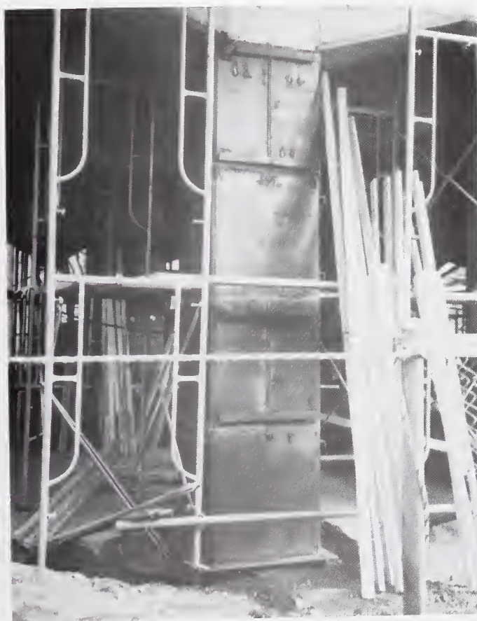
Figure 4.3.8 Jacketed column - JR Main Line.
