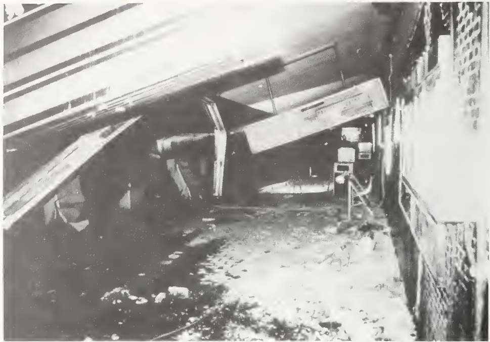
Figure 4.3.19 Roof collapse viewed from the station platform at Daikai Station.
