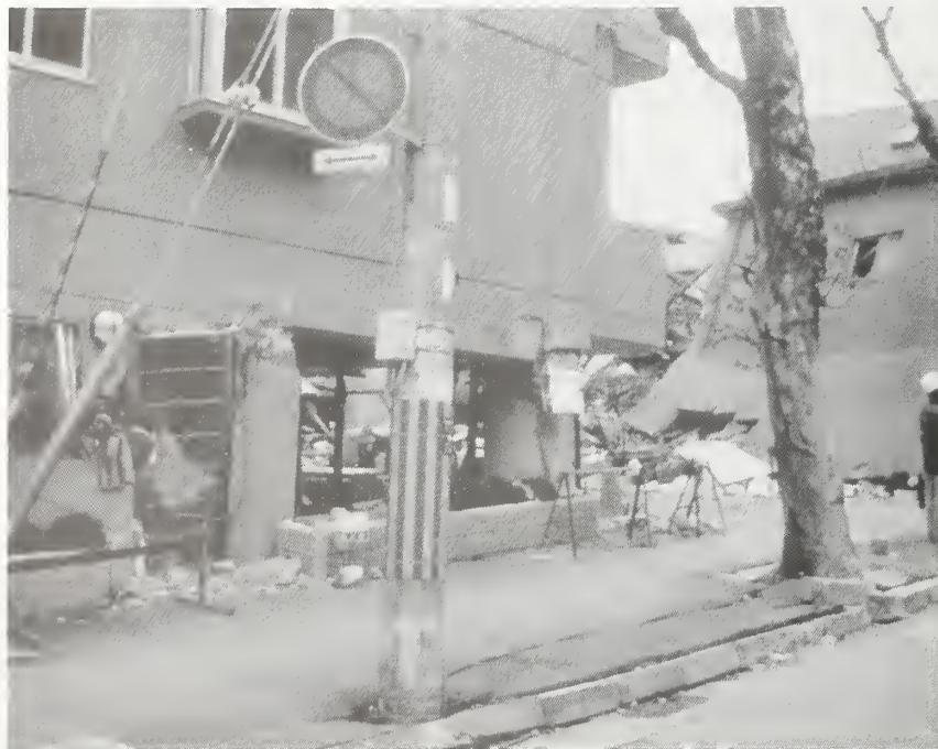
Figure 3.4.14 Collapsed first story near JR Line.
