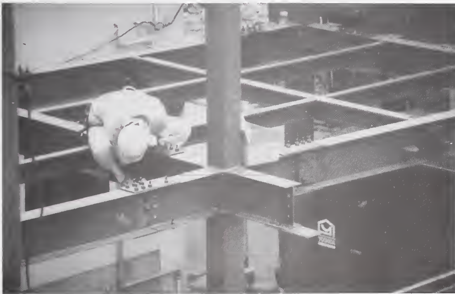
Figure 3.5.2 Field joint assembly of prefabricated steel frame structure east of Kobe using all high strength bolted connections. Beam stubs, approximately 0.5m in length, are shop-welded for quality control improvement.
