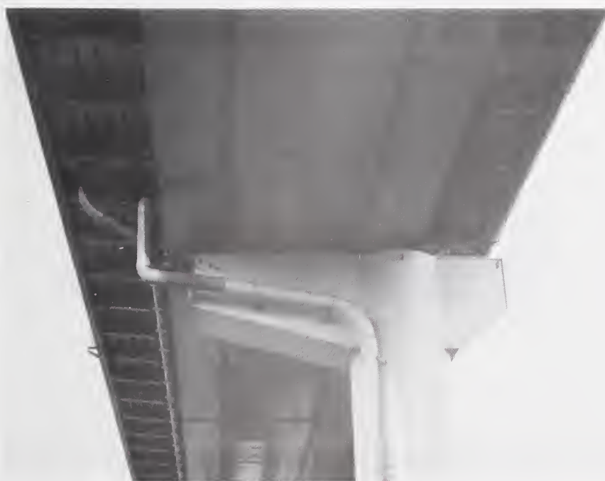
Figure 4.2.38 Failed bearings and lateral offset at top of Pier 586 of westbound Route 3.
