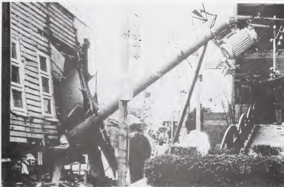
Figure 5.4.68 Fallen housed pushed over some distribution poles.
