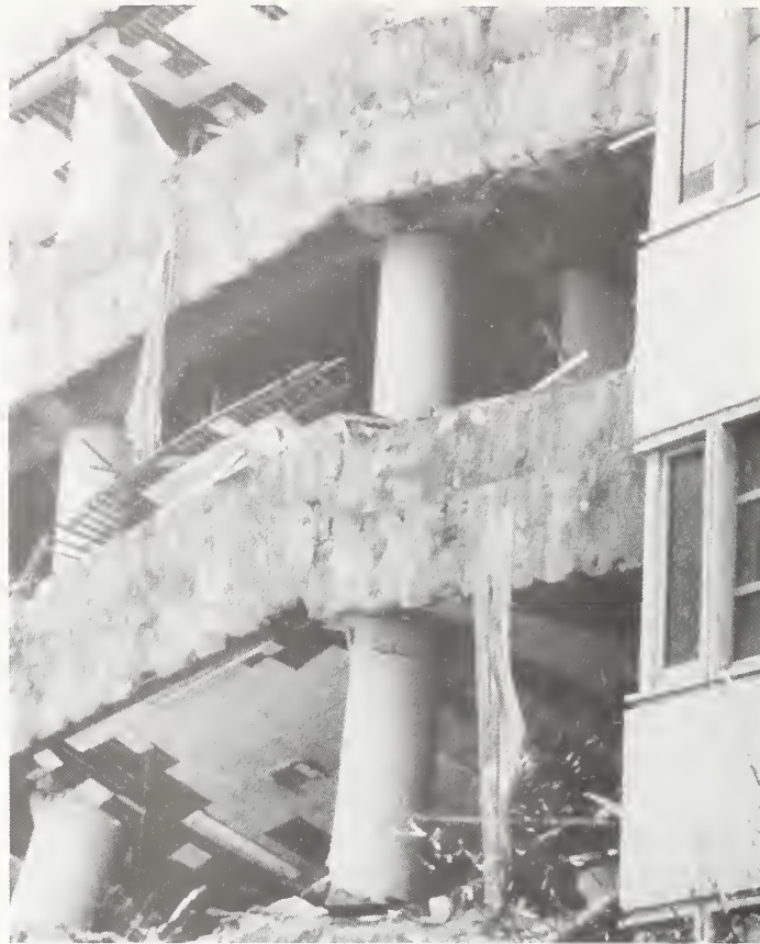
Figure 3.4.13 Strong beam-weak column failure.
