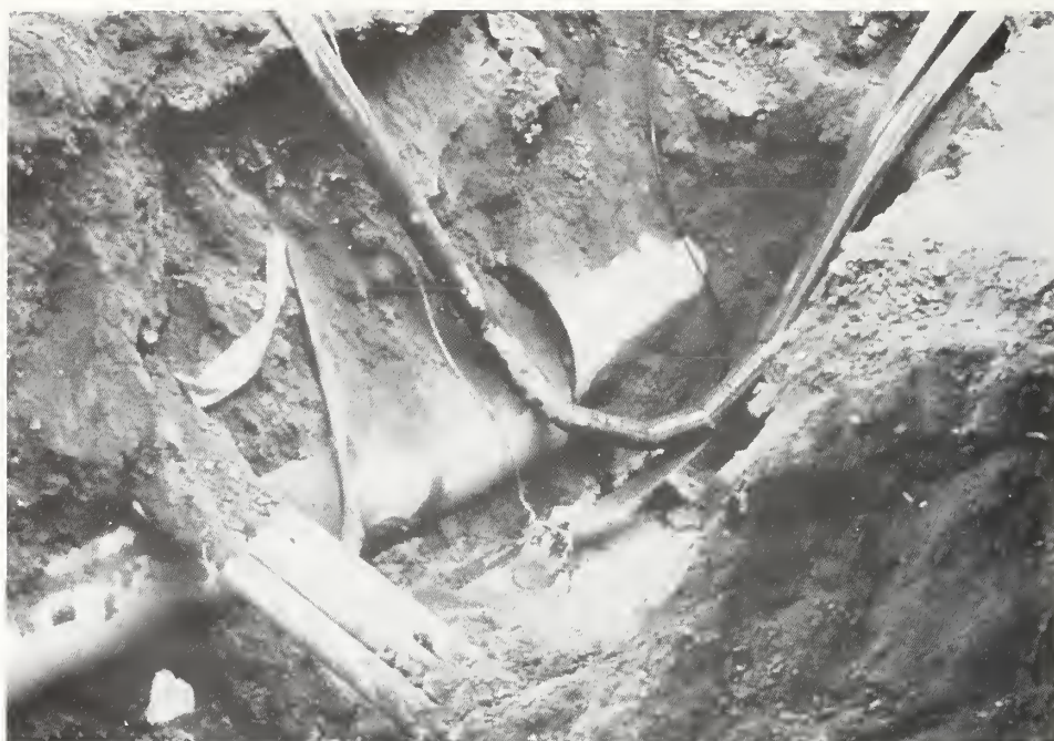
Photo 16 Repair of 700-mm welded steel pipeline which ruptured at a weld on the north side of Port Island in an area affected by liquefaction induced lateral spread. This line carries the entire potable water supply for the island.
