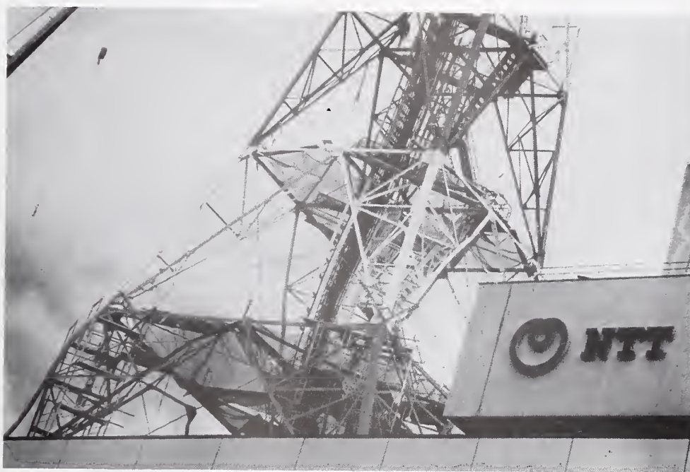
Figure 5.5.1 Microwave tower on top of a central office which was damaged and later removed.
