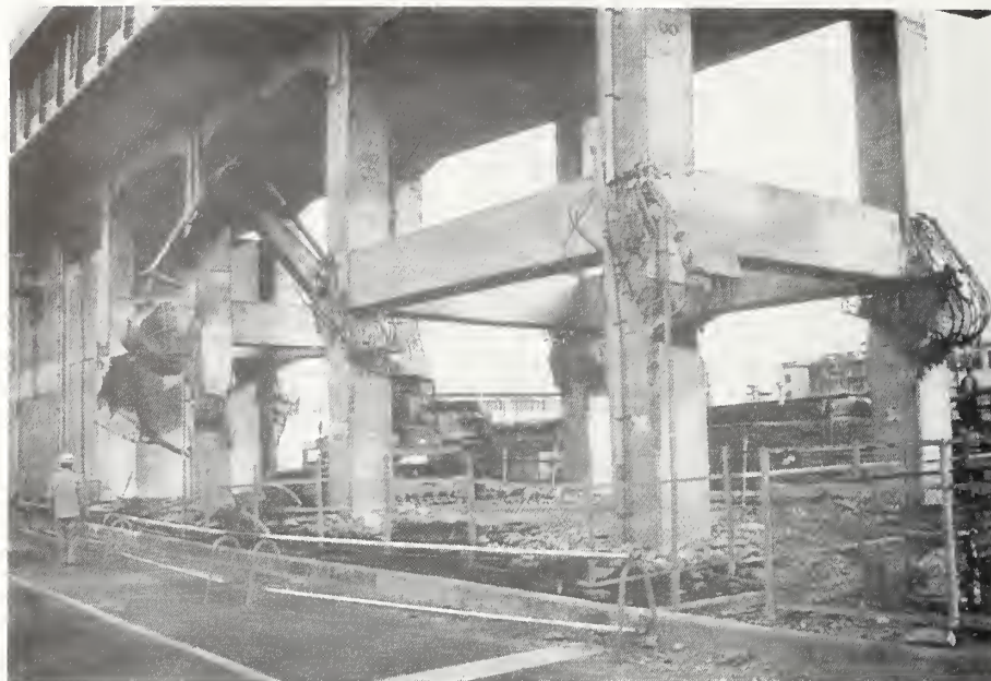
Figure 4.3.5 Damaged concrete frame - Shinkansen.
