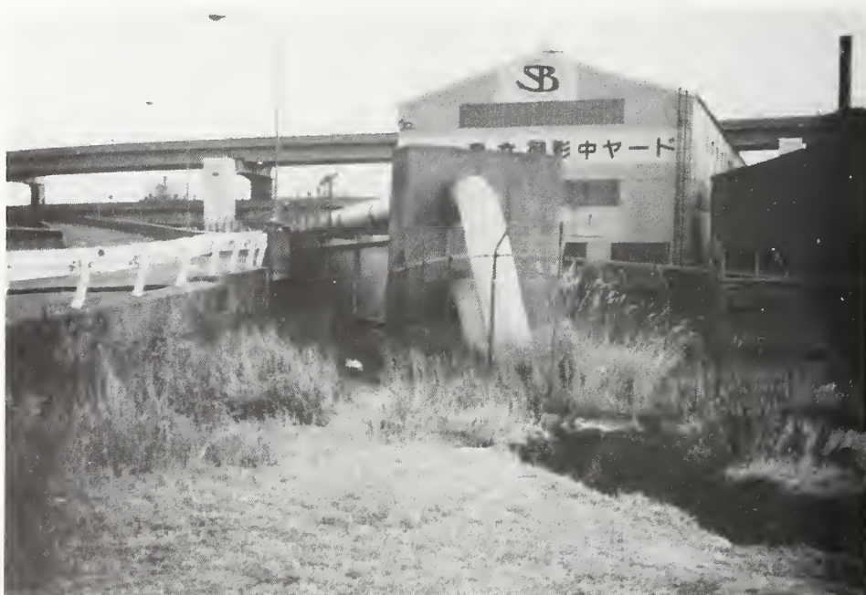
Photo 17 Ground cracking from lateral spread in fill area along a water way. Immediately behind the crack, a pipeline emerges out of the ground to be supported on the bridge.
