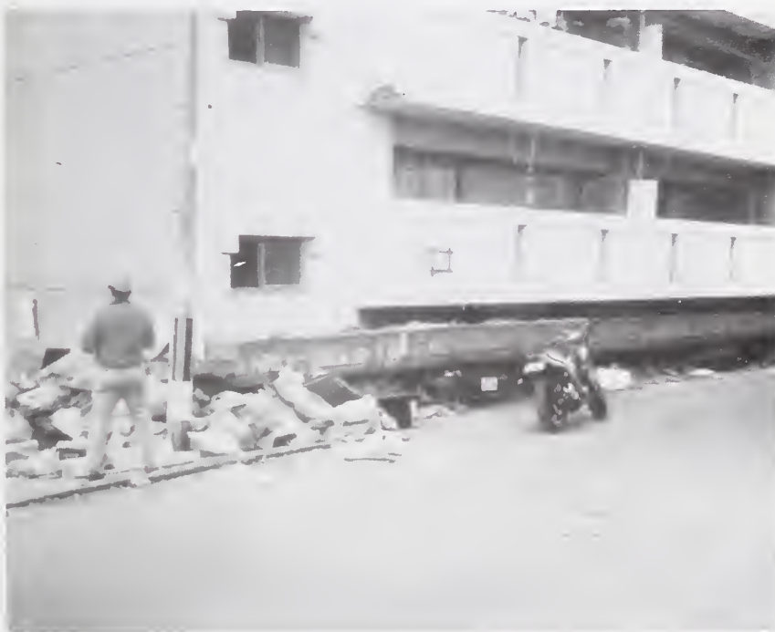
Figure 3.4.5 Failed ground floor shear wall - apartment building.
