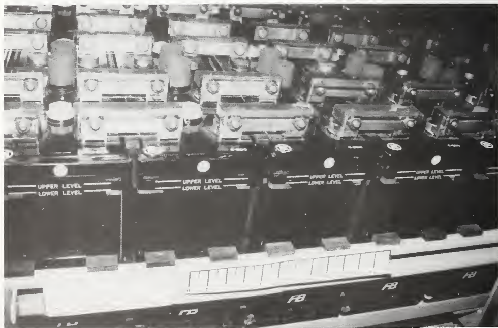
Figure 5.4.41 A different approach using rubber spacers in Japan to restraining cells to battery racks.
