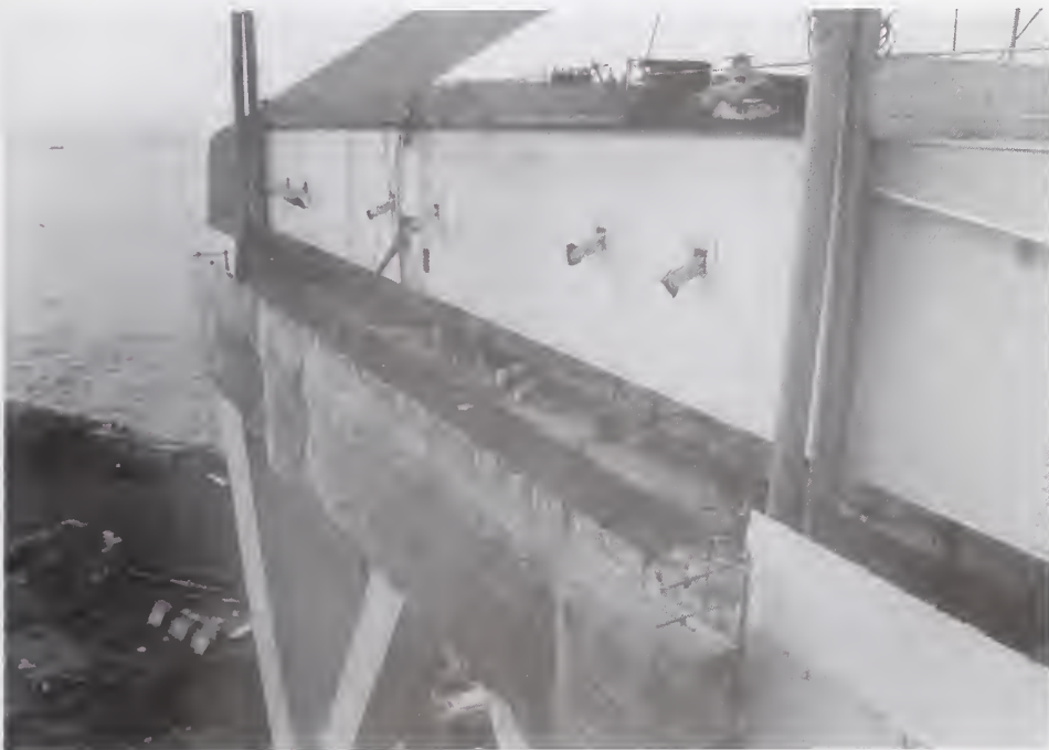
Figure 4.2.4 Cap beam of Pier 111, Nishinomiya-ko Bridge, showing cross-girder of arch and failed restrainers.
