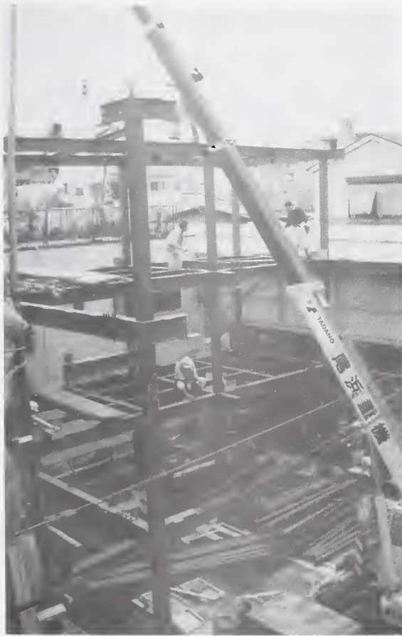
Figure 3.5.1 Typical modern 3 story new steel frame building being erected near Hanshin Expressway #3 east of Kobe. Columns are pre-fabricated so that no field welding is required.
