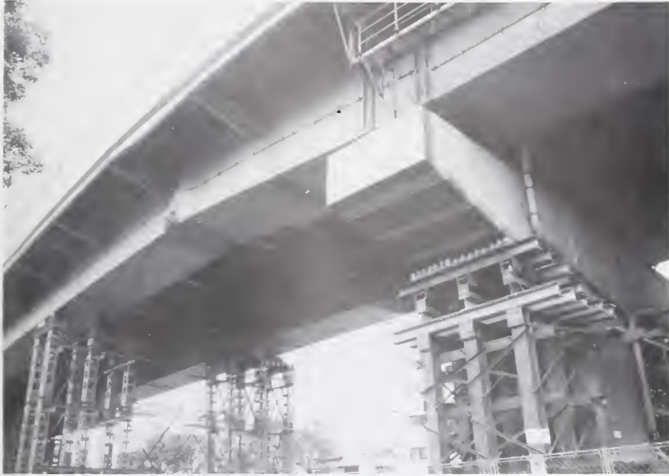
Figure 4.2.20 Compressive failure in lower flange of steel box girder between Piers 238 and 239 of Hanshin Expressway.
