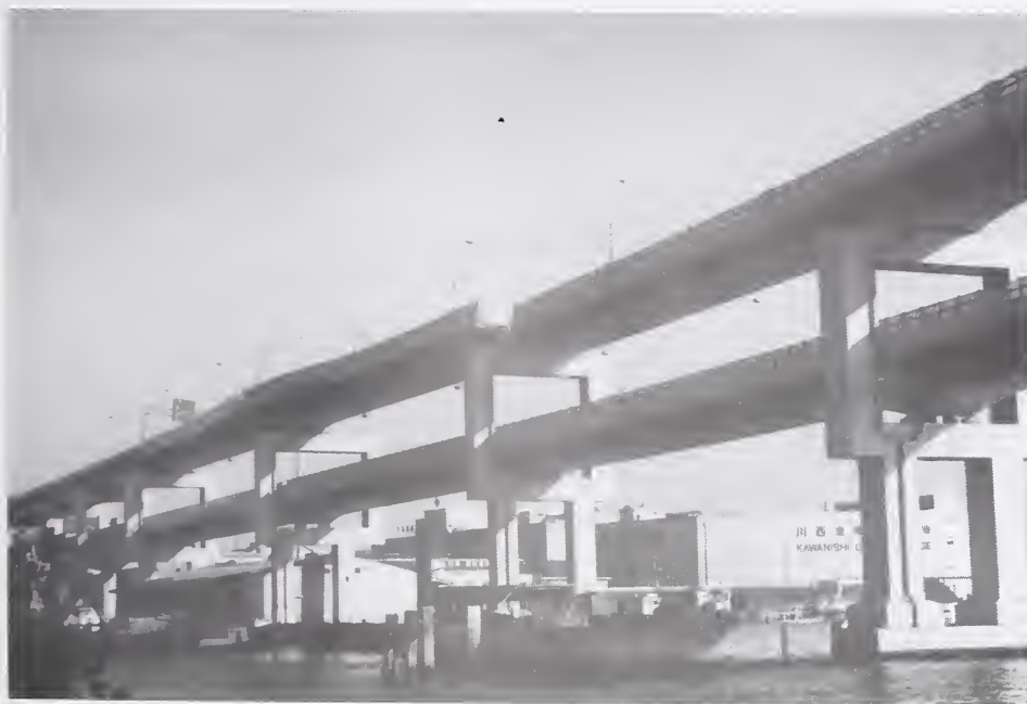
Figure 4.2.13 Lateral offset at Pier 36 in upper level of Hamate By-Pass due to bearing failures at Piers 34 through 38.
