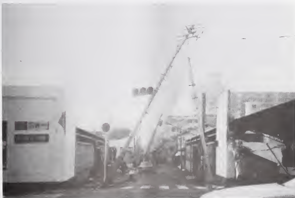
Figure 5.4.69 Some poles failed due to inertial loads or were pulled down by other fallen poles.
