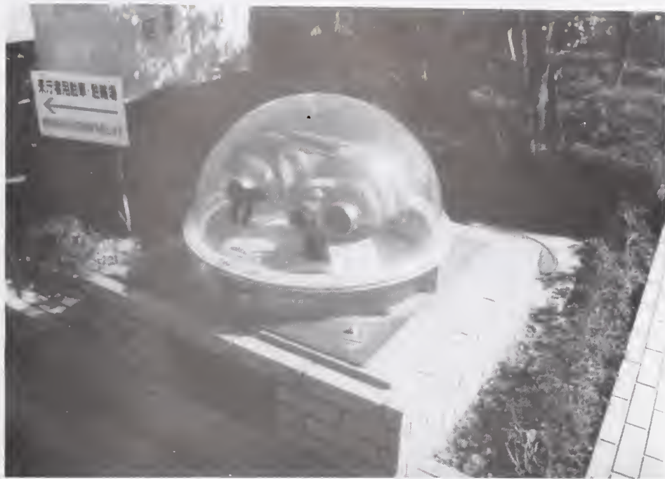
Figure 6.2.21 Seismically reinforced fire fighting water cistern.
