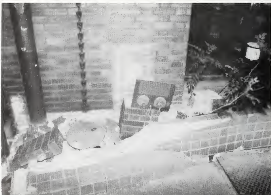
Figure 6.2.12 Standpipe connection severed at street level.
