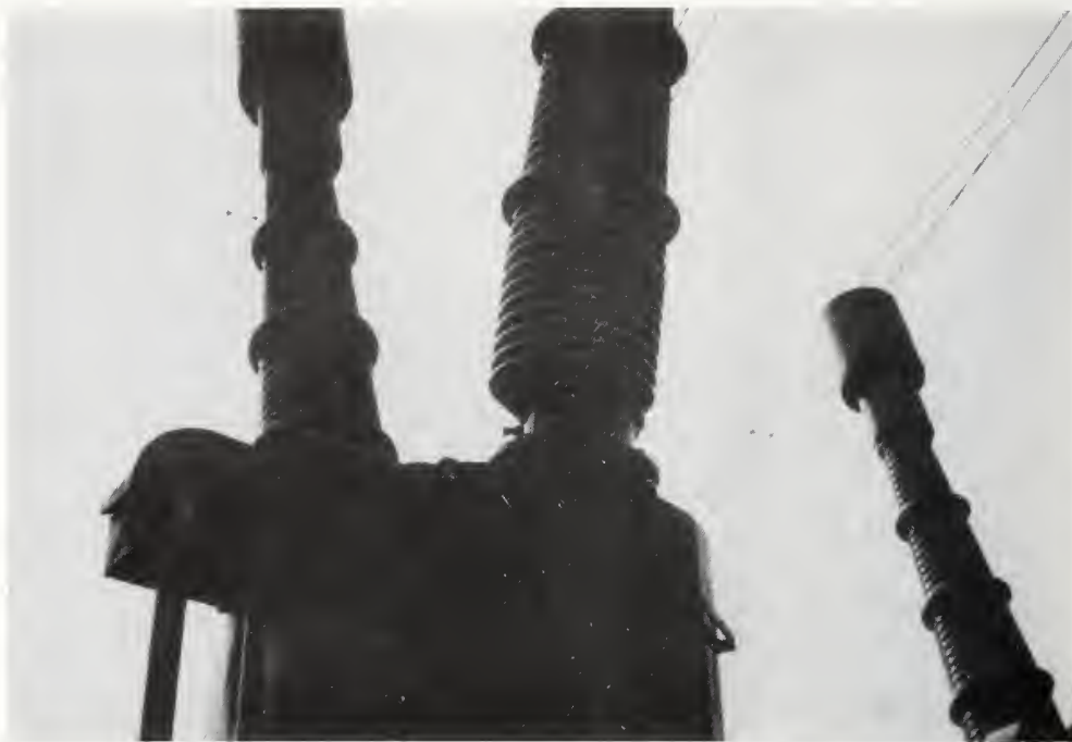
Figure 5.4.25 The porcelain slipped on its lower flange on a 275 kV bulk-oil Circuit breaker.
