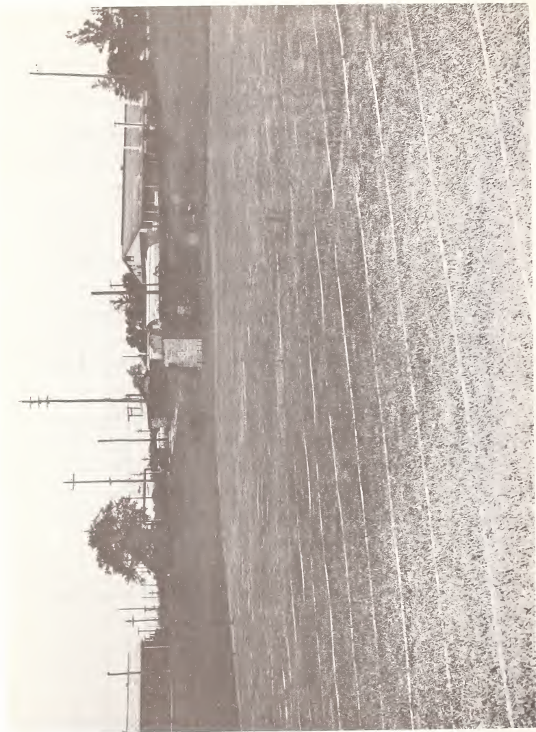
VIII.16 Photograph of First Concrete Blockhouse Built at the U.S. Army Chemical Center to Study Structure Shielding.
