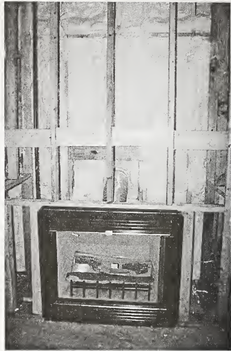
Foam insulation applied around the direct vent propane fireplace.
