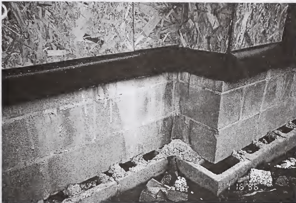
Figure 2: A detail of the Huntsville Health House showing the water drainage sheet.
