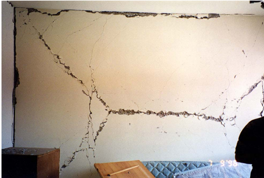
Figure C22. Interior wall exhibiting yield line damage
