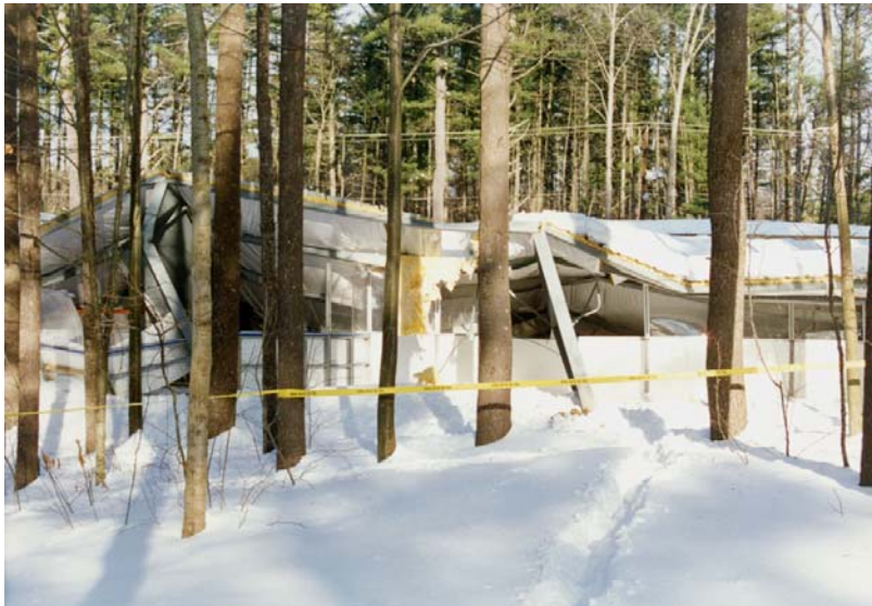
Figure C8. Collapsed Jackson Landing Skating Rink
