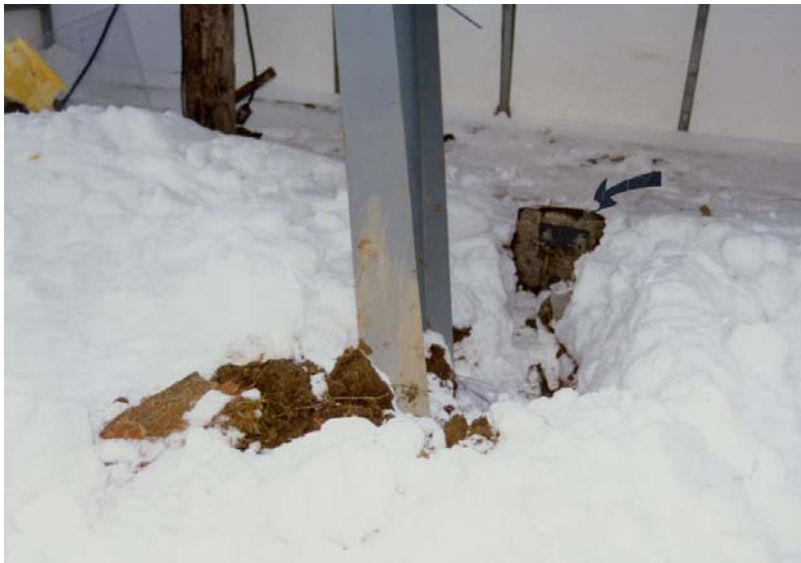
Figure C11. Split pier (arrow) at failure initiation location
