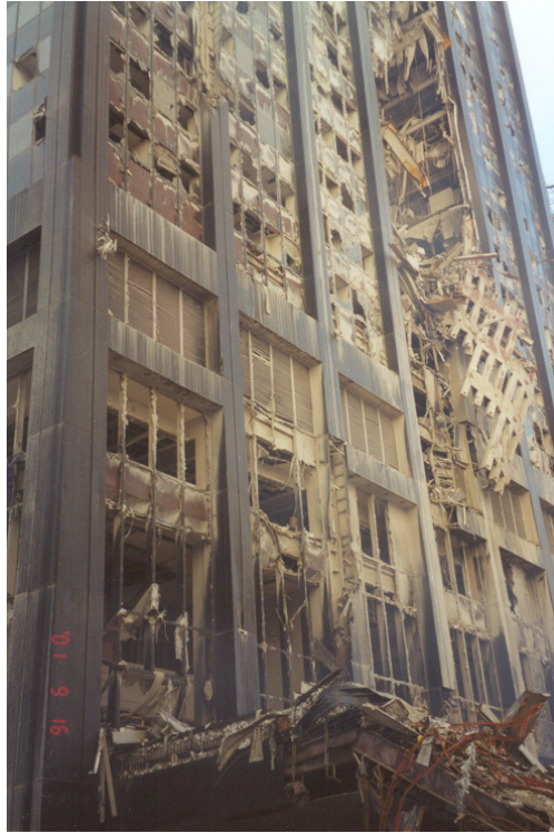
Figure C16. Gash in North Face of 130 Liberty Street
