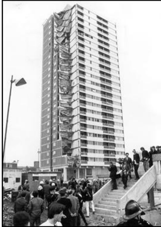
Figure C1. Ronan Point after collapse
