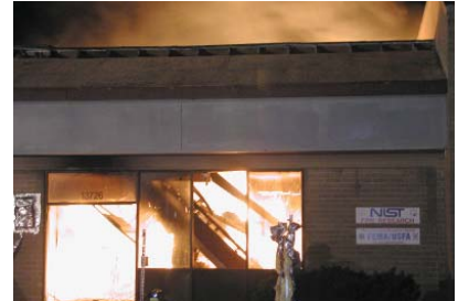
Roof collapses in shopping center store fire.
