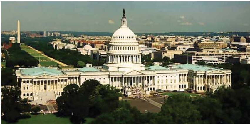
BFRL researchers are assisting the architect of the Capitol in the design, installation, and operation of a BACnet System.
