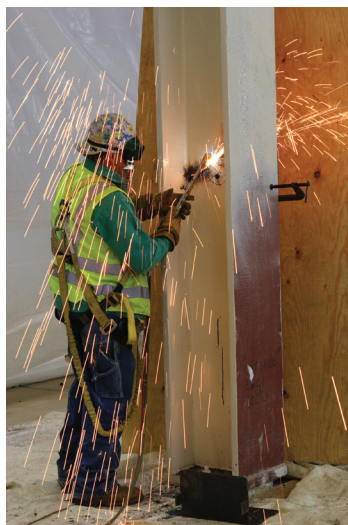
And it didn't come tumbling down: removing the final columns between the guide hall east and west wings.
