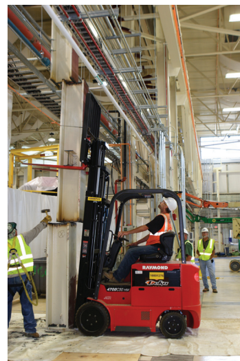
And it didn't come tumbling down: removing the final columns between the guide hall east and west wings.
