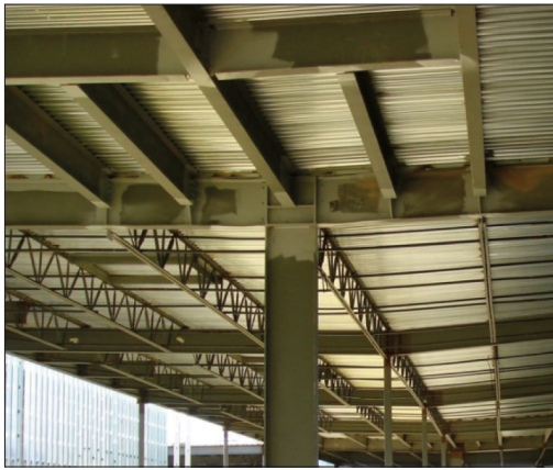
Figure 5-2. Stability bracing using transverse framing.
