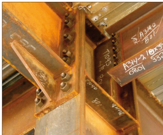
Figure 7-2. Installed connection continuity plates in a bolted stiffened extended end plate connection.
