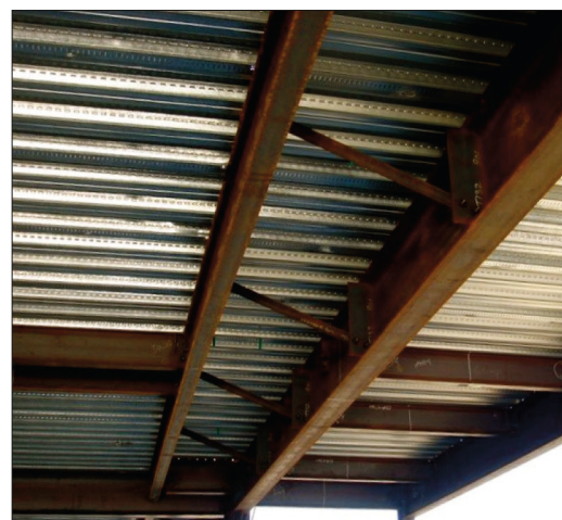
Figure 5-1. Stability bracing using diagonal “kickers”.
