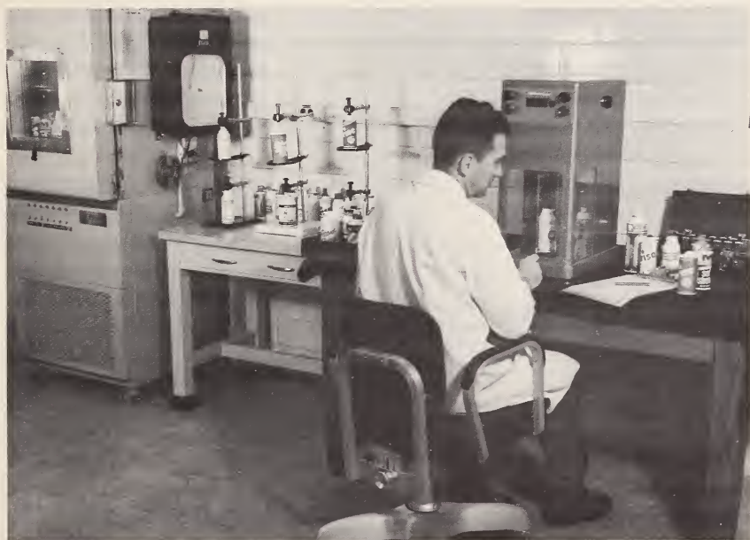
Weighing aerosol cans during a research program to establish effective test procedures for determining net content of aerosol products. (See page 171)
