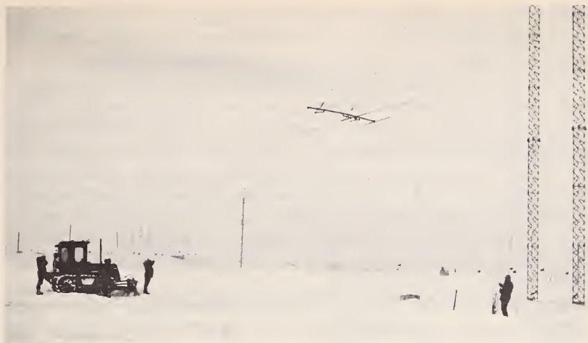
Raising antenna at the South Pole Station for the detection of solar proton events by VHF forward scatter observations. This program is a cooperative effort by U.S., British, and Russian scientists. (See page 217)
