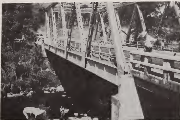
Figure 33 CA9-Teculutan - Typical Through Truss
