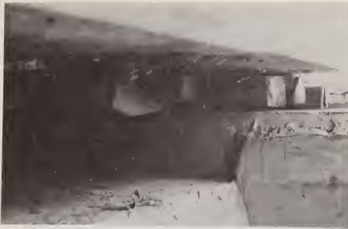
Figure 30 Incienso' - Missing Neoprene Bearing Pad at South Girder, West Abutment
