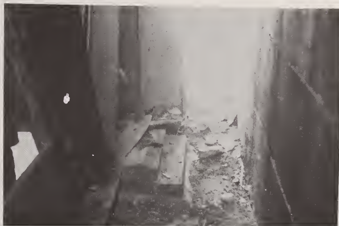
Figure 20 LaAsuncion - Displaced Girder, East Abutment
