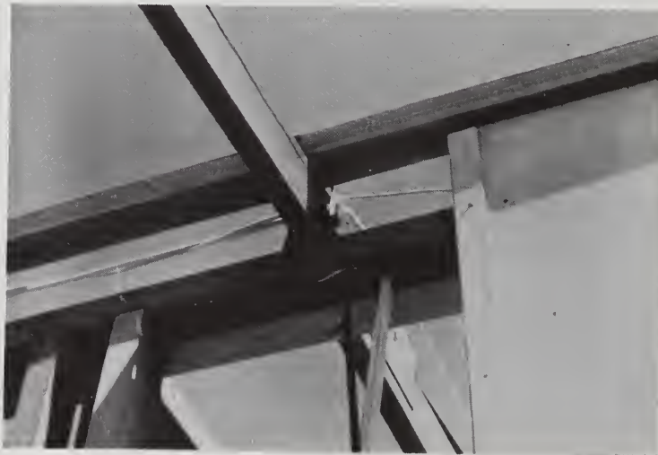
Fig. 8. Cyclone bolt and rafter connection
