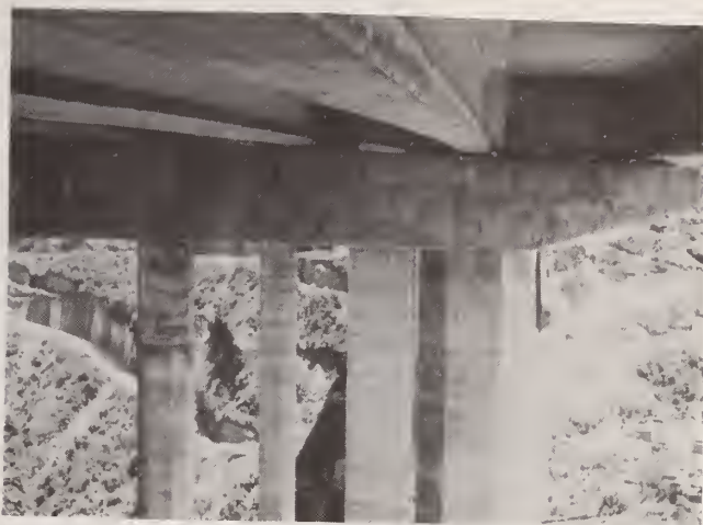
Figure 27 Incienso - Hinge Restraint, West Pier Bent
