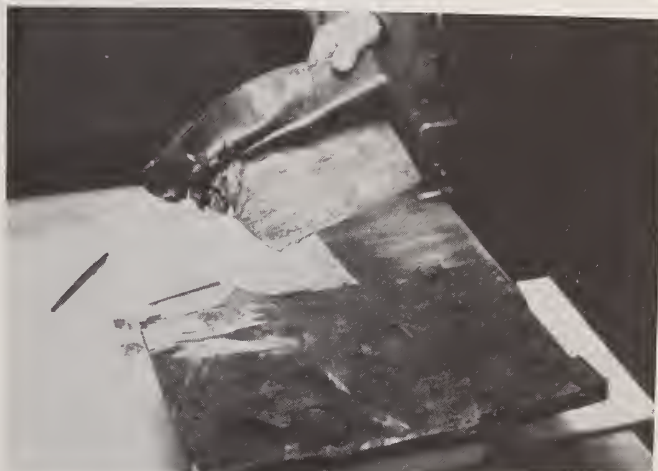
Figure 29 Incienso Dislodged Neoprene Bearing Pad
