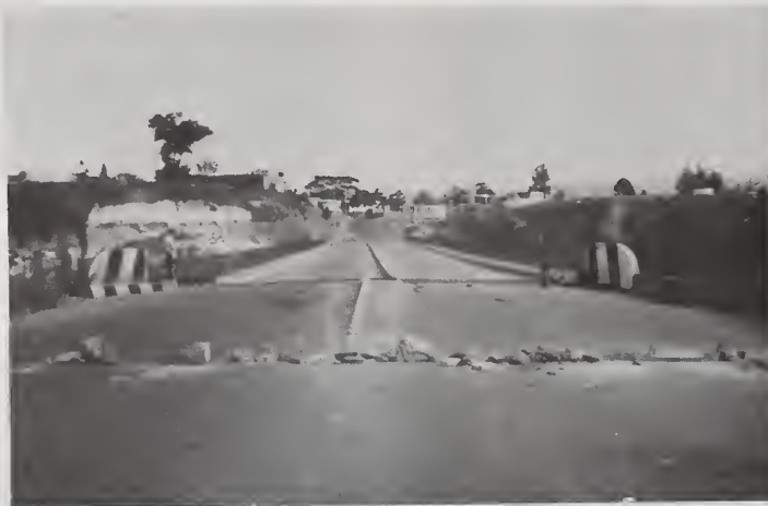
Figure 14 LaAsuncion - Lateral Offset at West Abutment
