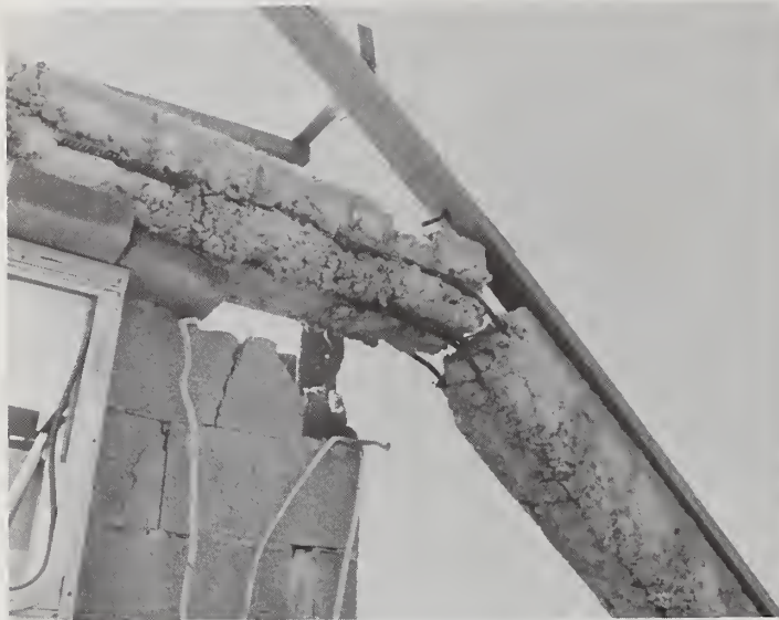
Fig. 11. Concrete bond beam and timber plate (single-story construction)
