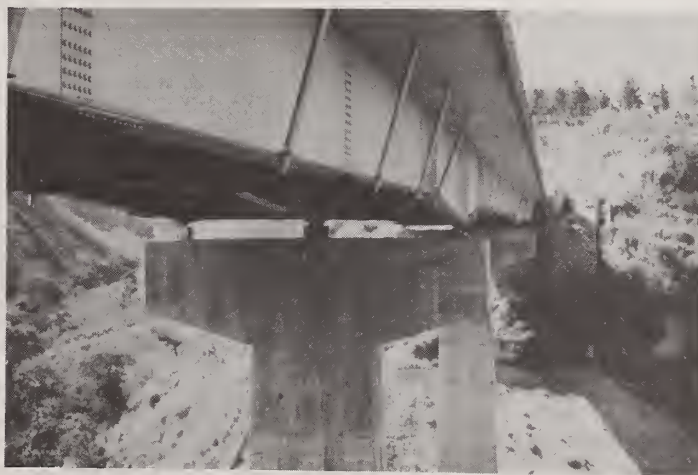
Figure 21 LaAsuncion - Missing Bearing, East Pier
