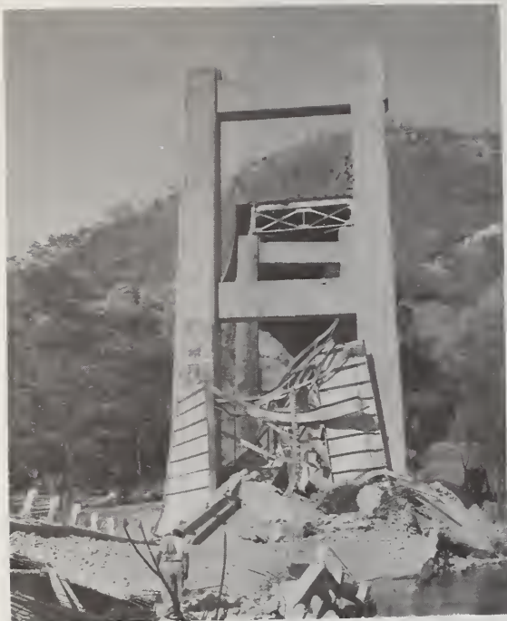
Figure 6 Agua Caliente Collapsed Center Span and Roadway
