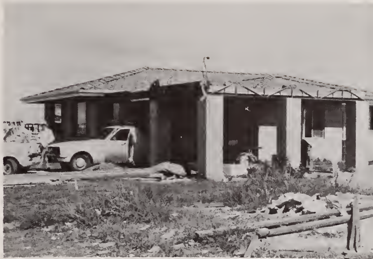
Fig. 17. Privately constructed residence with welded steel frame and brick veneer
