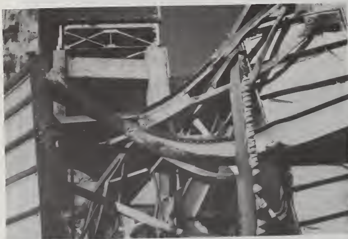
Figure 7 Agua Caliente - Detail of Collapsed Span at Base of Pier 3
