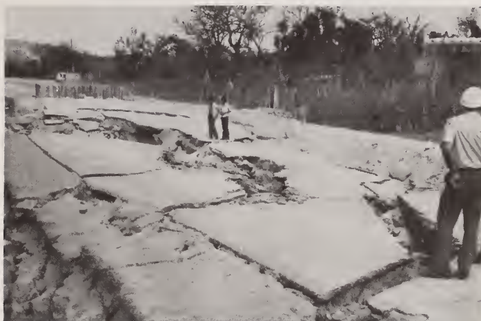
Figure 35 CA9-Typical Road Failure
