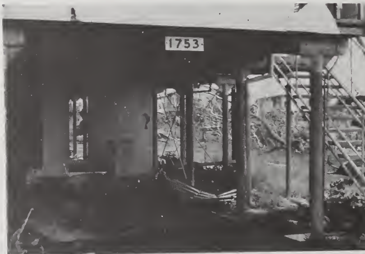
Fig. 4. Pipe columns used in older construction
