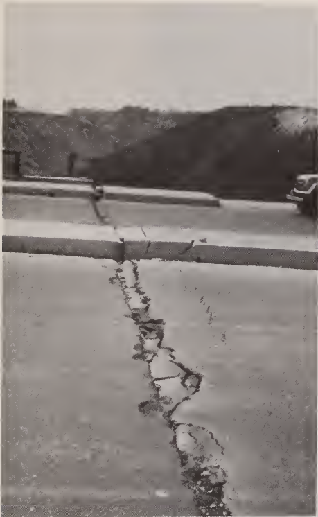
Figure 25 Incienso - Pavement Cracking at West Abutment
