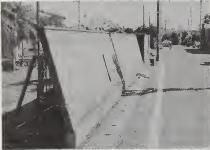
Photo-18. Damage of concrete block fence
