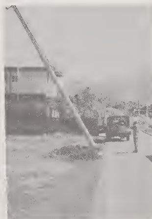
Photo-17. Damage to telegraph pole
