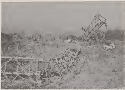
Photo-12. Damage to guyed tower (on top of Mt. Mihara)
