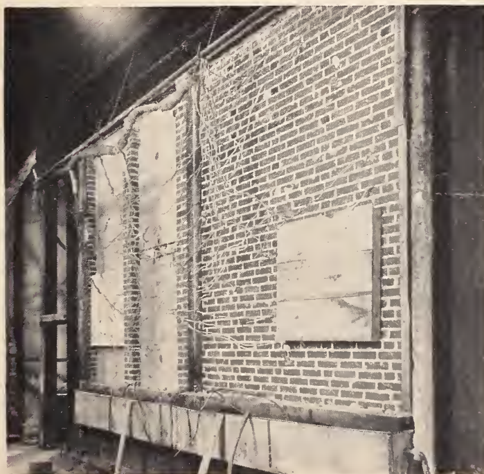
FIGURE 8. Unexposed side of walls 10A and 10B before test.
