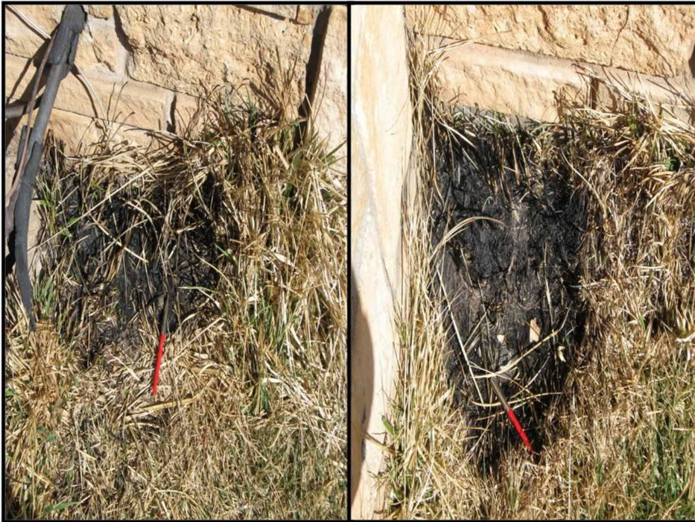
Figure 21 Two distinct vegetation ignitions adjacent to structure at 209 Quail Ridge Road. Red feature is 15 cm (6 in) long ballpoint pen, NIST photos.
