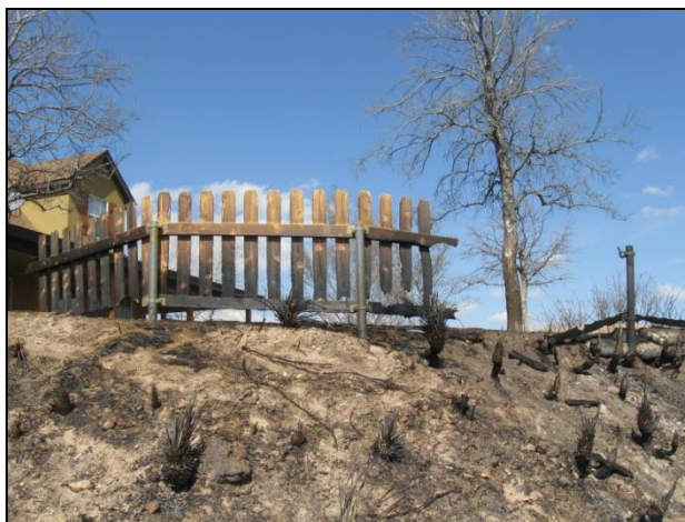
Figure 54 Partially destroyed fence at 100 Camino Alto, NIST photo.
