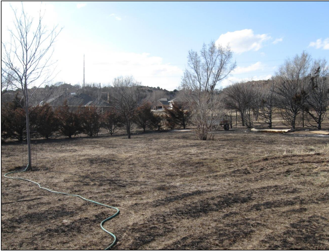
Figure 58 Burnt hedgerow and Buffalo grass that facilitated fire spread to destroyed secondary structure at 105 Port-O-Call Drive, NIST photo.
