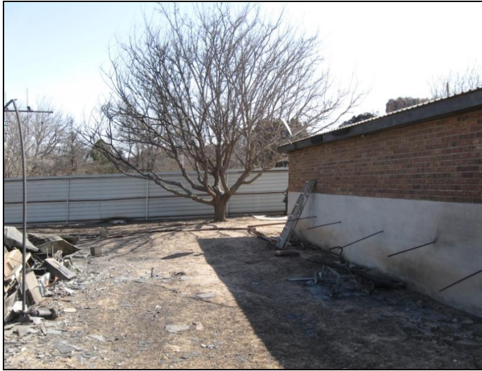
Figure 34 Unidentified burned features adjacent to the northern side of the residential structure at 102 Gary Drive. These features are believed to be ignited by the burning mobile home to the north of the brick residential structure, NIST photo.
