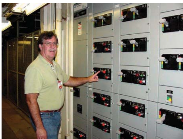
FIGURE 1: Operations Electrical Engineer Dennis Brady inspects the status indicator on a newly installed Motor Control Center.
