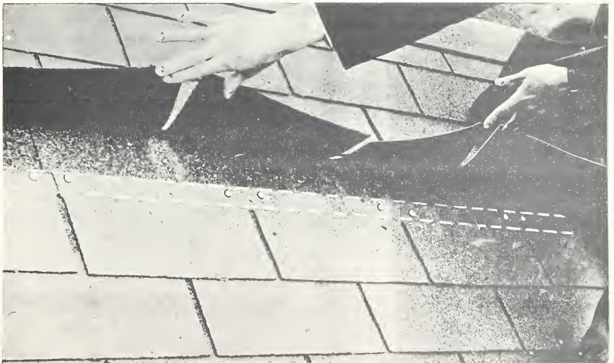
Figure 32. Proper nailing of asphalt shingles.
