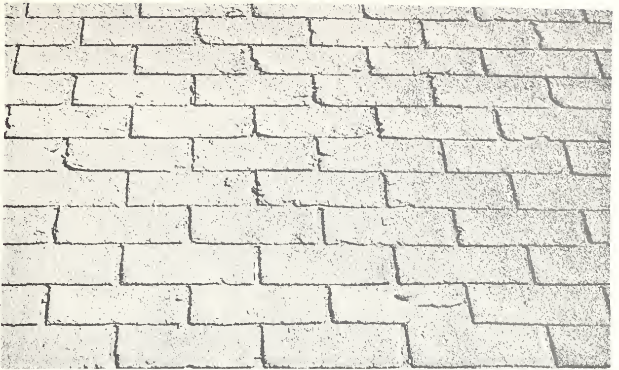
Figure 31. Recoated asphalt shingles. Note damage due to brittleness.
