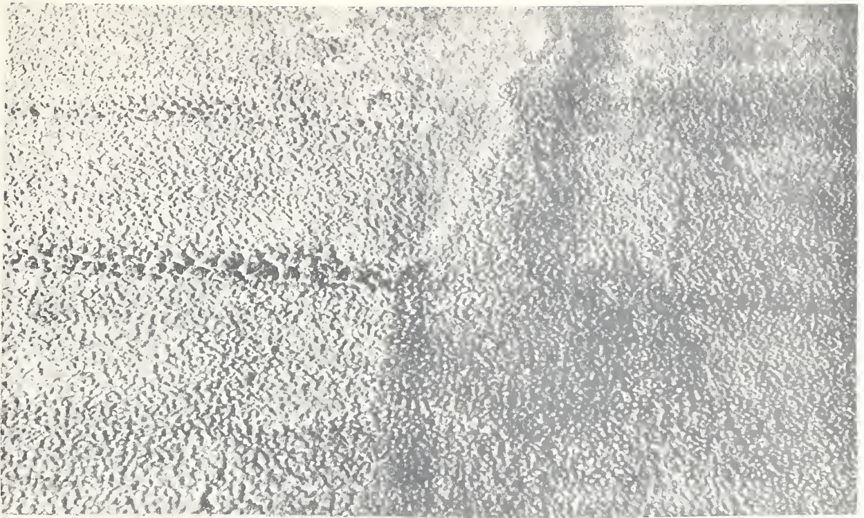
Figure 23. Comparison of cold coating (asphalt emulsion) with and without the glass membrane.
