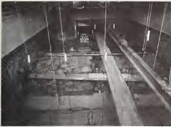
FIGURE 7.—Top of floor for standard fire test, showing asbestos pads covering surface thermocouples, deflection measuring tapes, and method of loading with pig iron.
