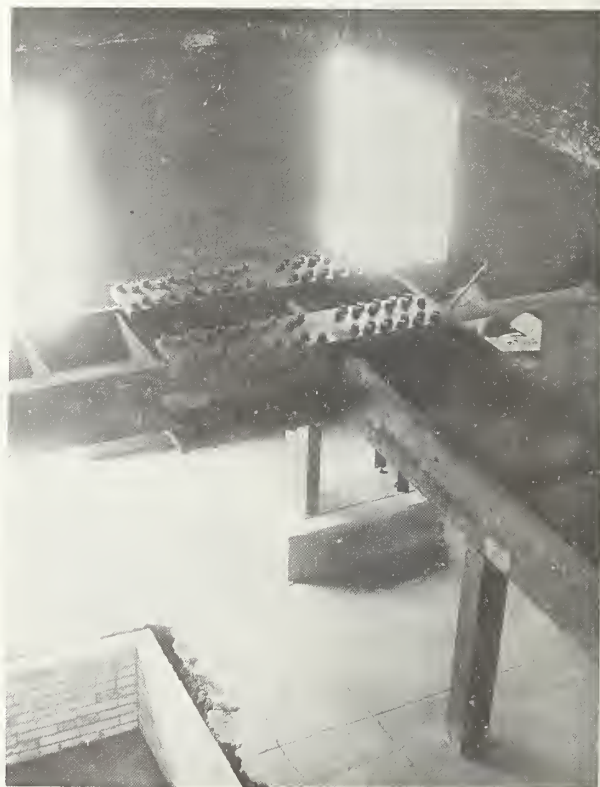
FIGURE 2.—Floor test furnace during construction; corner fastening and column supports visible.
