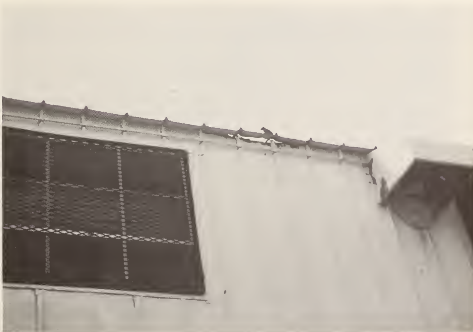
Figure 3. Illustration of loss of metal at top edges of panels under the eave
