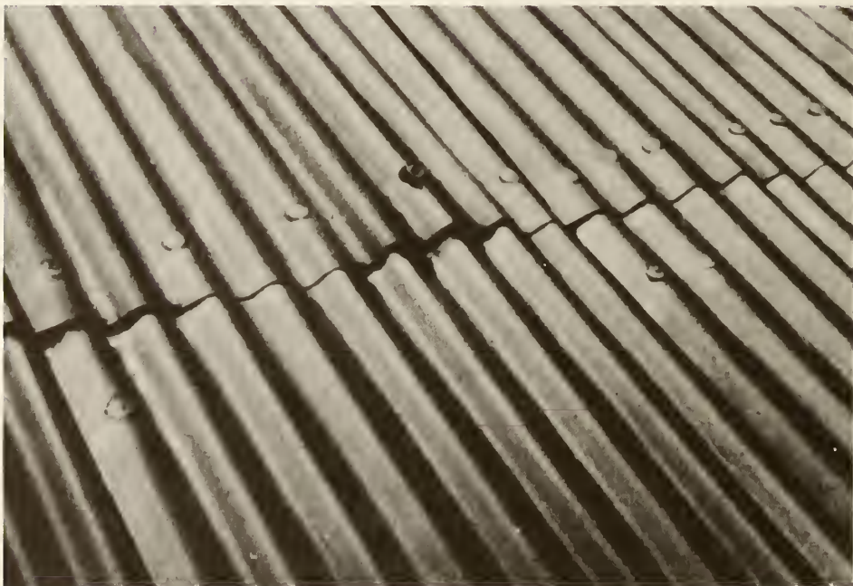
Figure 11. Loose fasteners
