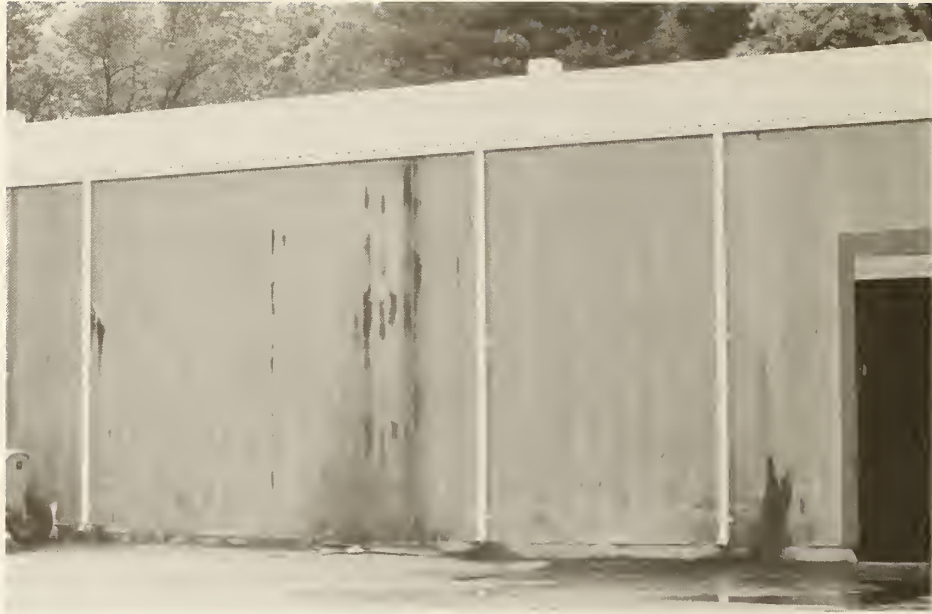
Figure 12. Corrosion of galvanized steel panels
