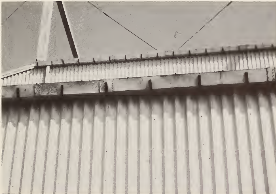
Figure 9. Corroded gutter hangers
