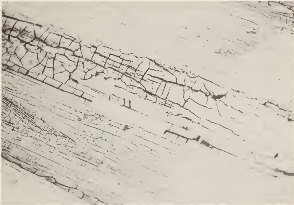
Figure 20. Severe cracking of bituminous roof coating
