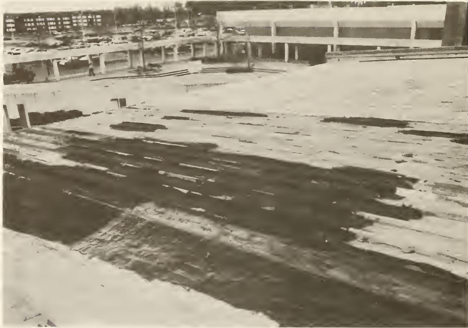
Figure 6. Thick fibrated bituminous roof coatings
