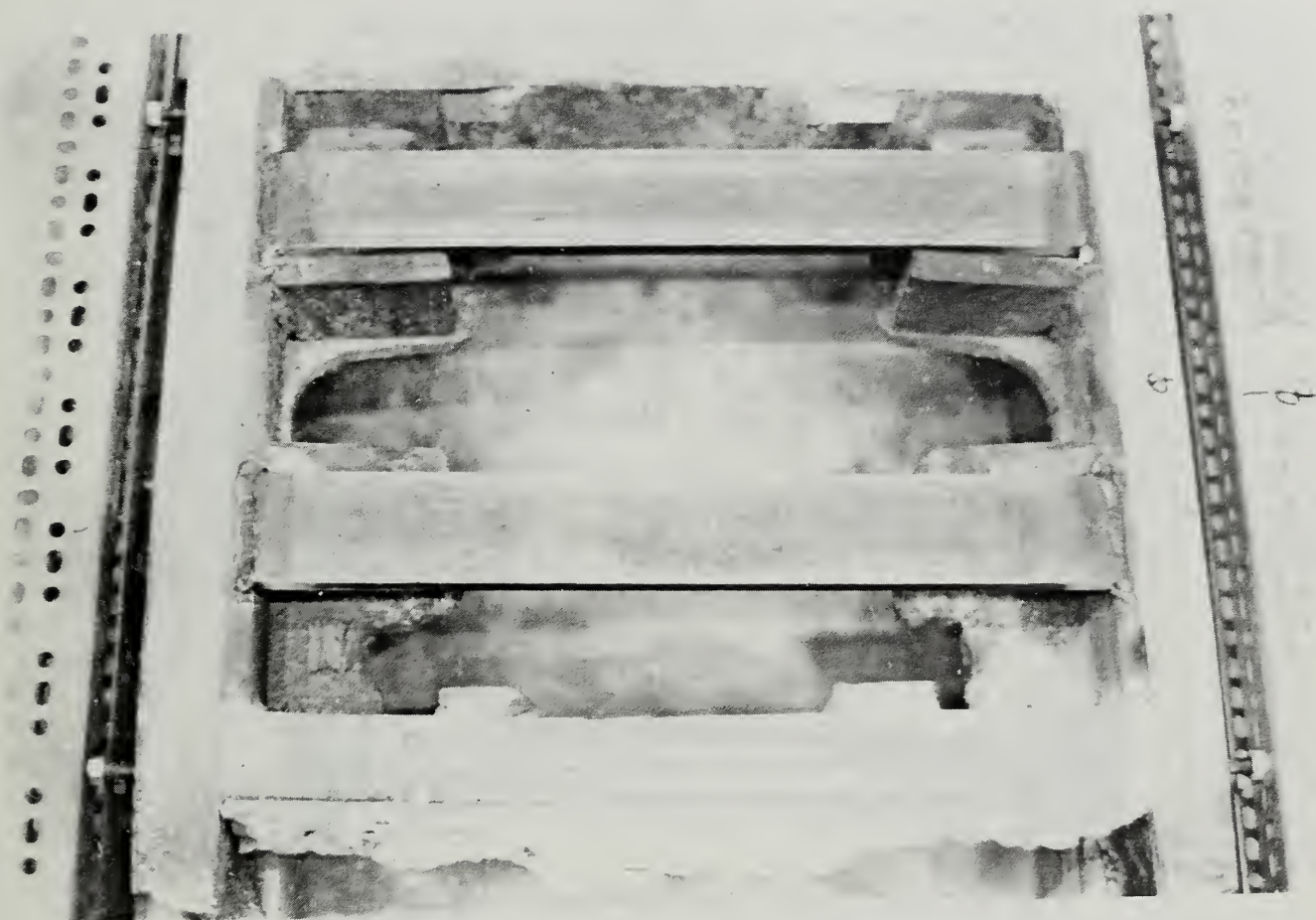
Figure 5.5.15 Shearhead No. 3 stiffened by plates welded between legs of lifting angles
