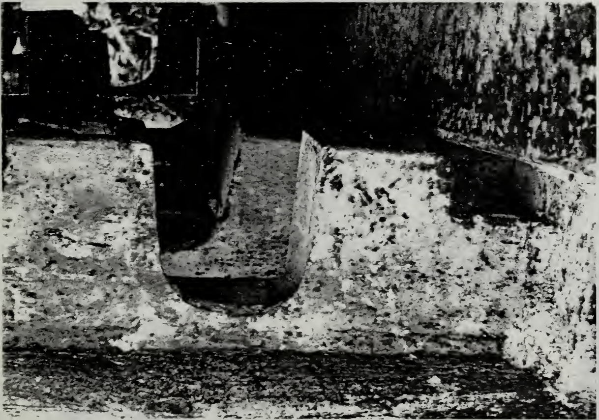
Figure 9.3.2 Indentations in underside of lifting angles, column E4.8, level 9
