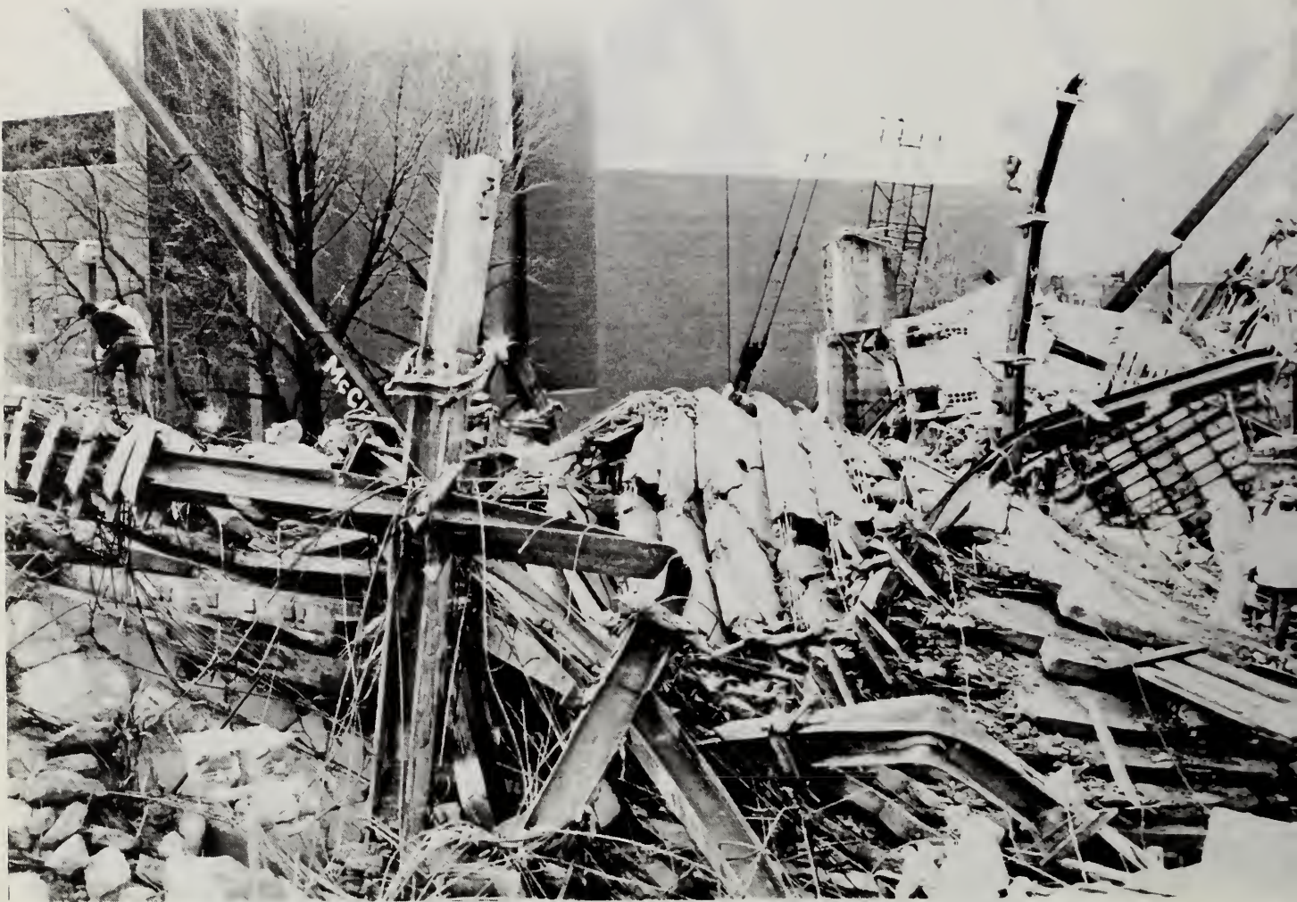
Figure 4.4.11 Floor slabs in the central portion of East tower – View to the Southwest
