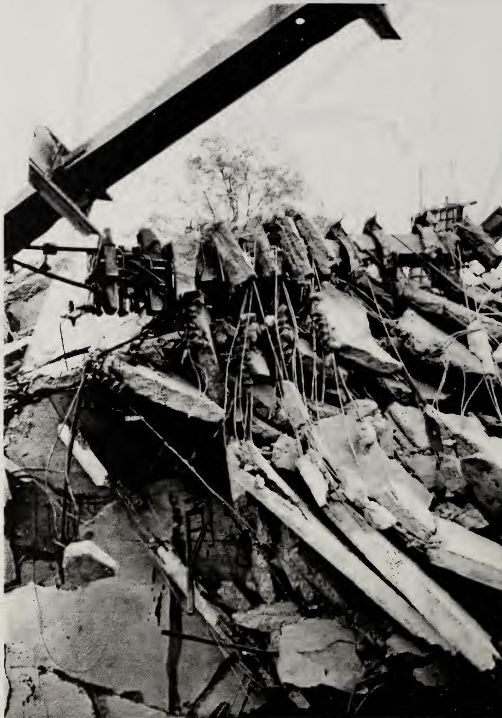
Figure 4.4.15 Separation of floor slabs from shearheads
