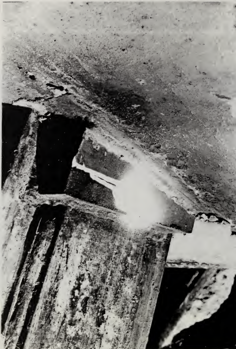
Figure 4.4.23 Intact shearhead support
