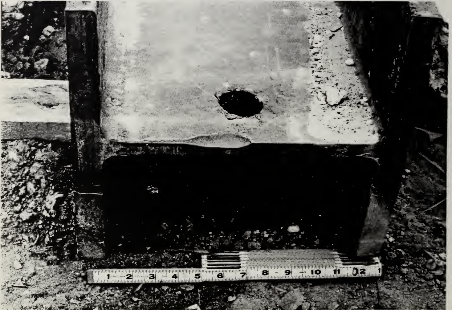
Figure 9.3.1 Indentation in top of column E4.8
