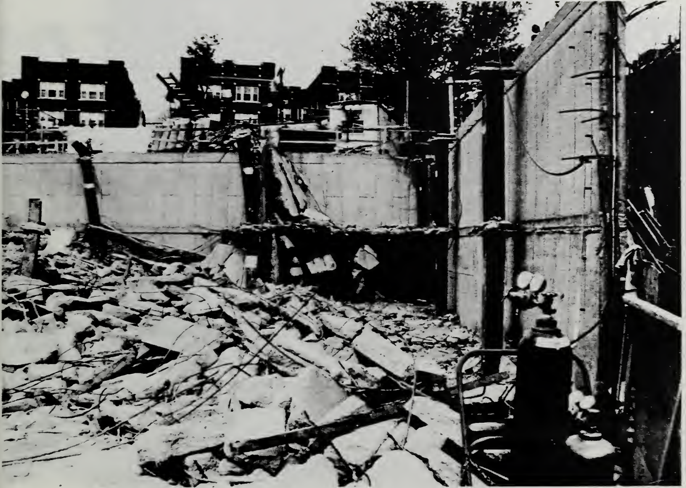
Figure 4.4.4 East perimeter columns at Levels E and D. East tower— View to the North; photo taken after rescue operations complete
