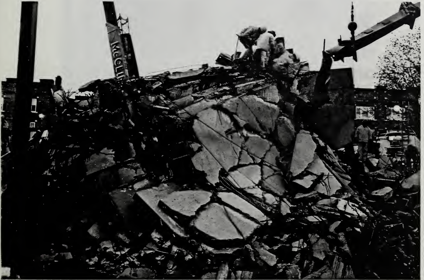
Figure 4.4.16 Floor slab crack pattern
