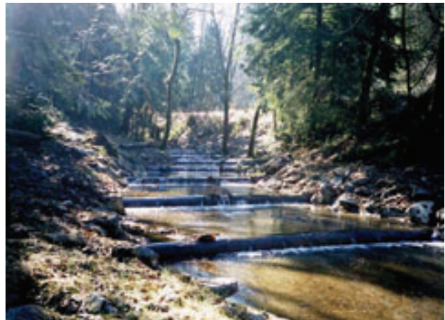
Figure 6 Step fishways can help fish move around a man-made barrier.
