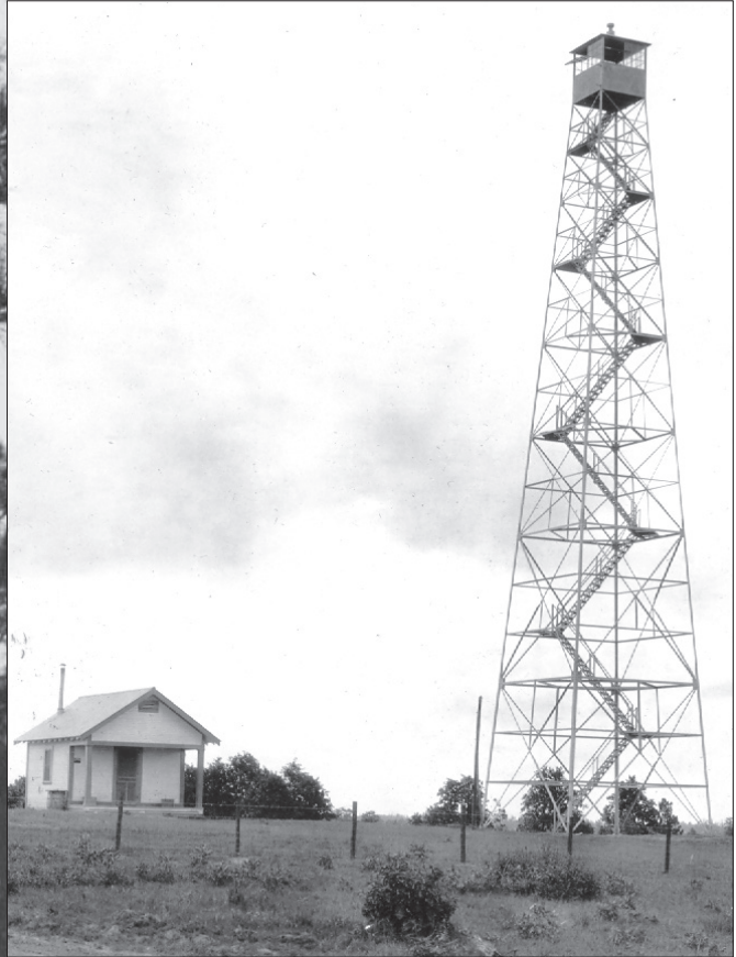
LEFT: A Civilian Conservation Corps worker climbs a pine tree to dislodge cones for seed collection. BELOW: This 100-foot steel lookout tower with cabin near Gardner was constructed by Civilian Conservation Corps enrollees of Camp F-3.
